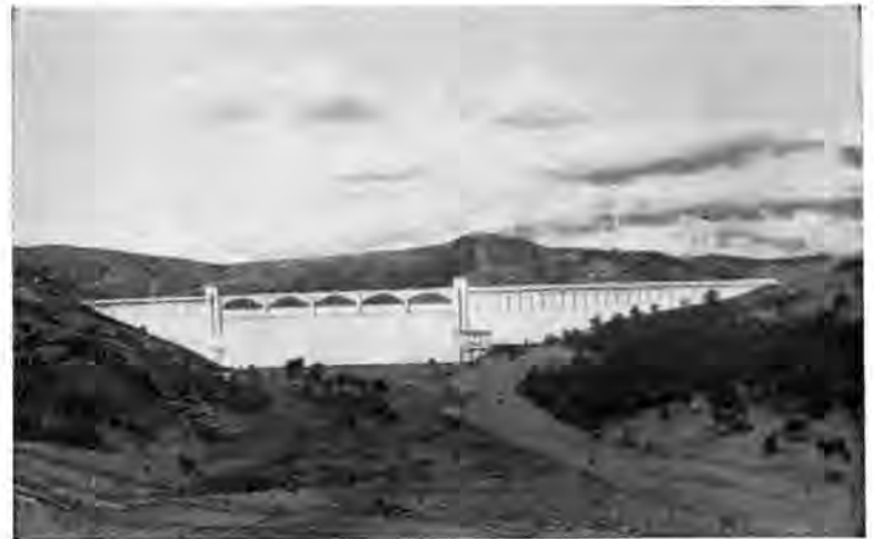
View of the dam from downstream, as it will appear when completed.
