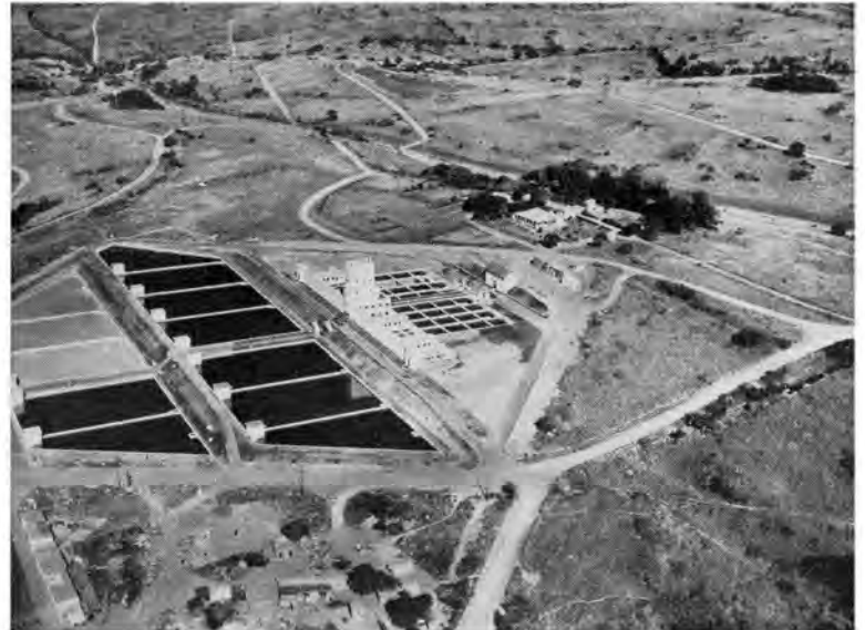
The Durban Heights water purification works, photographed from the air.
