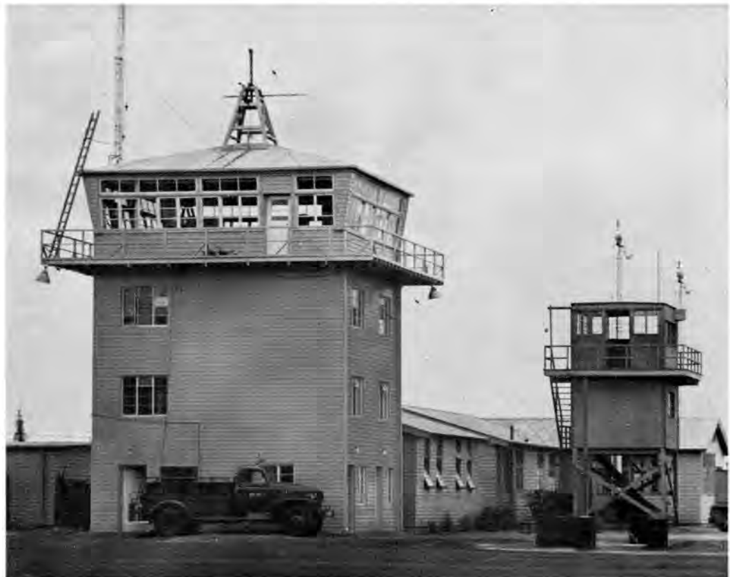
The new Control Tower at Palmietfontein Air Port, erected to meet the demands of the continually rising volume of air traffic. The old control tower is shown on the right of the picture.
