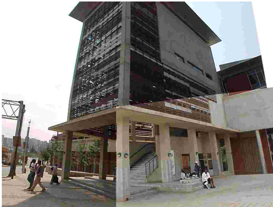
0 7 6 Metro Mall Main Entrance on the corner of Bree and West Streets
