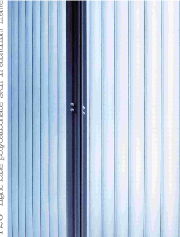
126 Light blue polycarbonate skin in aluminium frame
