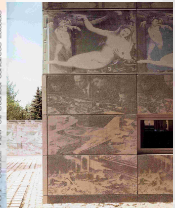
1.31 Corner view of etched concrete facade
