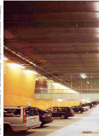
127 UN Studio's undulating expanded metal ceiling
