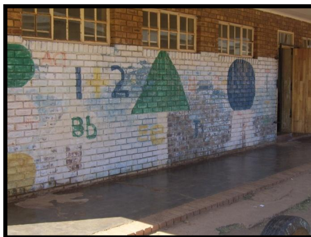
Figure 4.11: Neighbouring Primary School B (August 2010)
