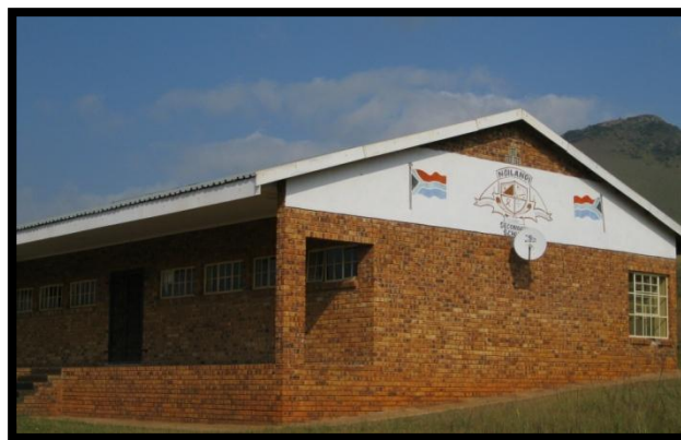
Figure 3.1: The main building of the selected rural secondary school (August 2009)
