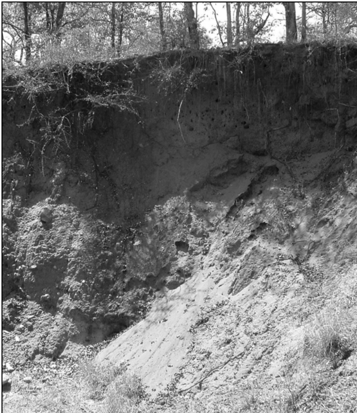
Figure 38: Sidewall of donga that cuts through BS04.
