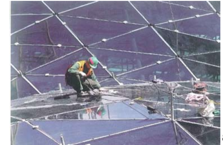
84 INSTALLATION OF GLAZING SEALANT
