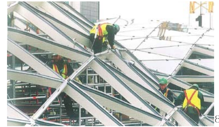
83 INSTALLATION OF GASKET SYSTEM
