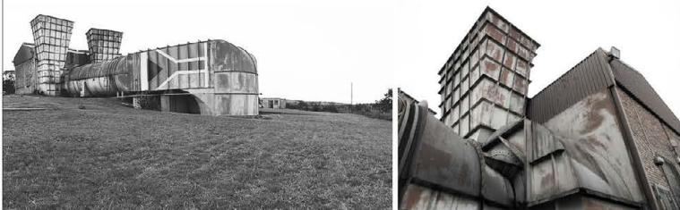
Mine ventilation shaft
