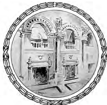
Figure 2.30 View of interior of Grand Foyer.
