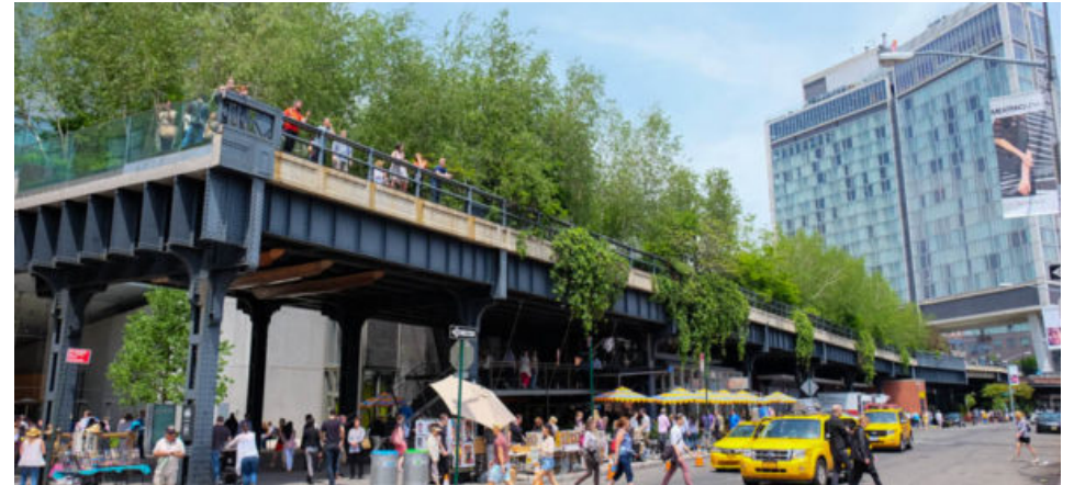
Figure.66: HIGHLINE ELEVATED PLATFORM (FIELD OPERATIONS 2009)
