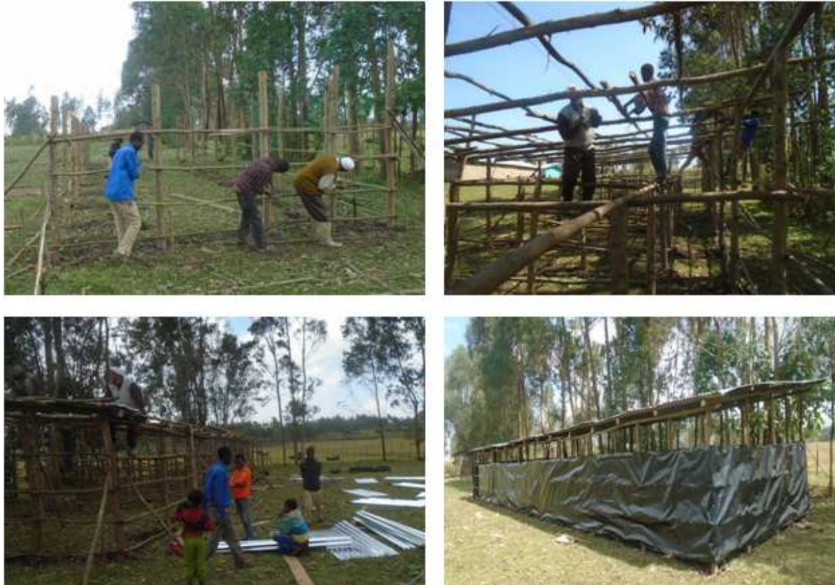
Plate 5.3. Partial view of experimental barn constructed at Gurmicho Primary School grazing land for controlled experiments during wet and dry seasons.
