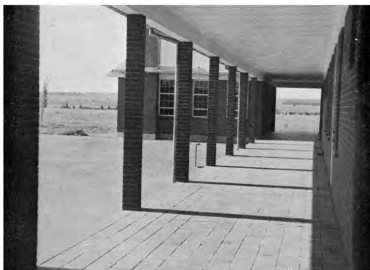
Vista along the colonnade on eastern side of main courtyard. A preparation room, laboratory, boys' lavatory, and cloakroom are to the right.
