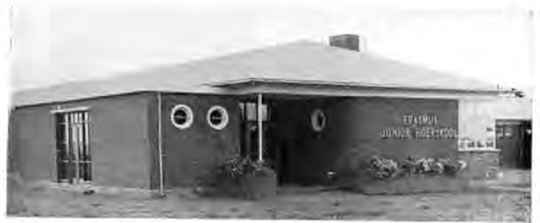
Entrance vestibule and Principal's office.
