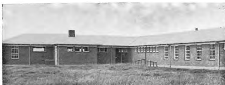
View from the south-west showing Domestic Science block on the left and girls' lavatories, preparation room and laboratory on the right.
