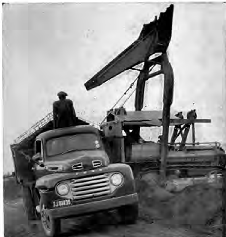
At work on the new Kempton Park airport—shifting soil with the Athey ML-4 Mobiloader.
