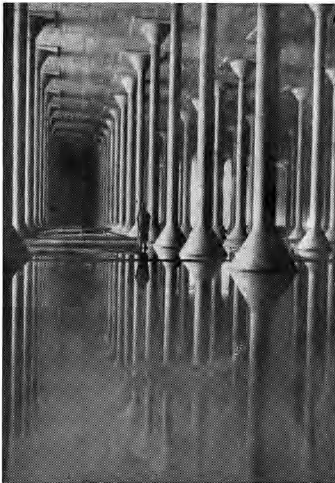
Interior of the Forest Hill Reservoir, completed in March, 1946. With an internal diameter of 395 feet, the capacity is 25 million gallons.
