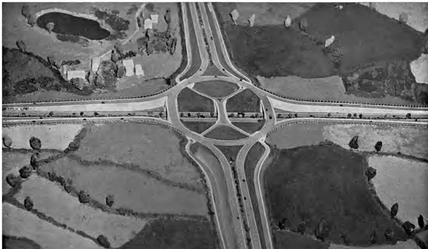
A road junction on one of Britain's new proposed "special roads." Fast traffic either way will continue at different levels while cycle and pedestrian lanes can also utilise the flyover at varying heights.
