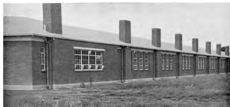
The south aspect. At the left is the Arts and Crafts centre, with the classrooms extending along to the right. Heating is by single-flue slow combustion stoves.
