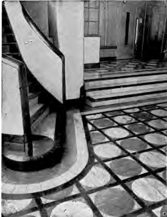
The entrance hall and stairs at Warrington Hall. This floor is made of 3/16" Press-cured Rubber Tile, laid on Supertox Rubber Compound.
