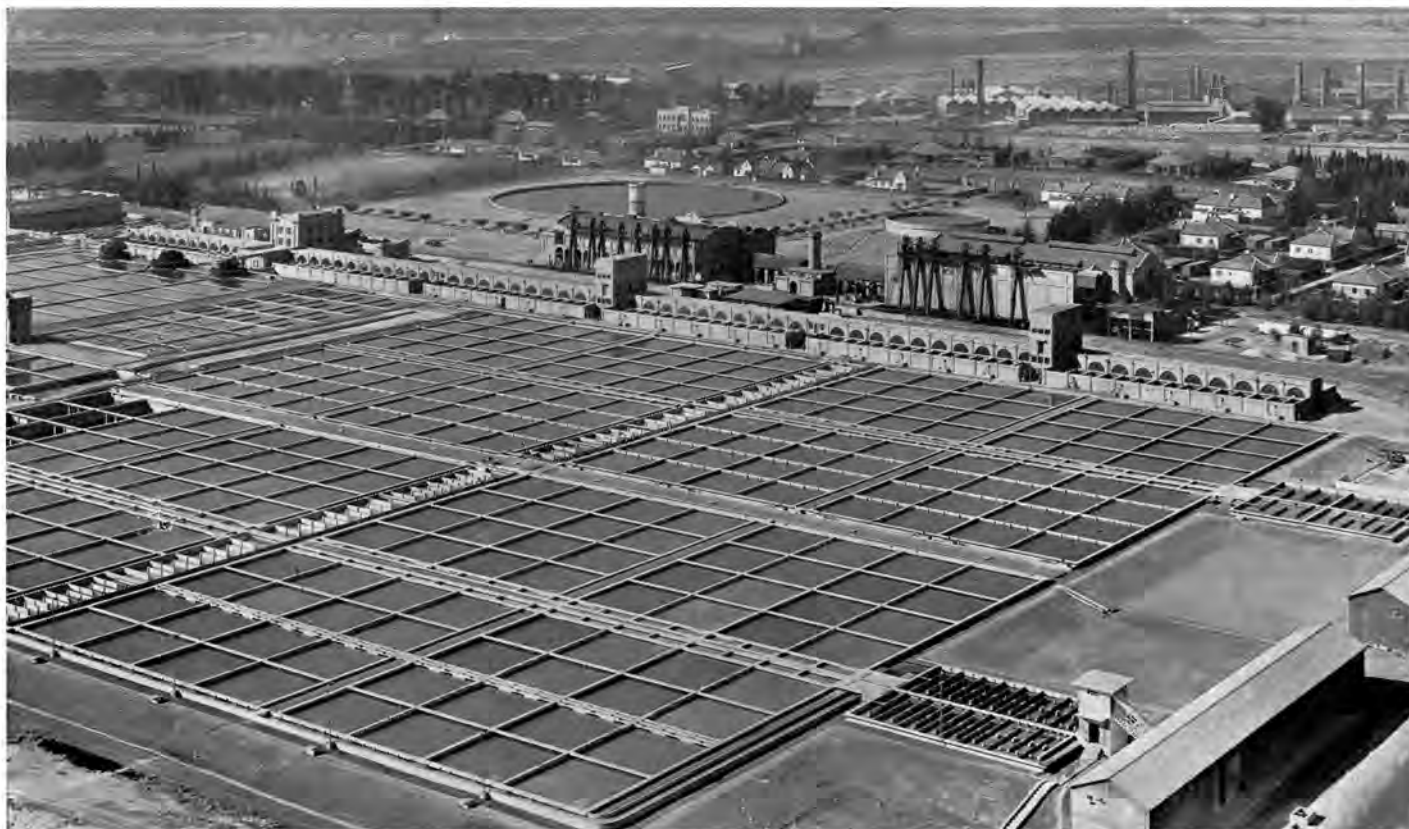
The Vereeniging Pumping Plant.
