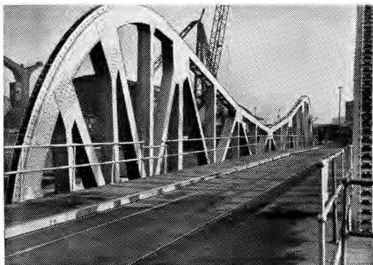
Sunderland's aluminium alloy bridge, the first of its kind in the world, and which cost £85,000 to build. The bridge, which weighs only 54 tons, spans a 90-foot wide junction between two docks and will carry road and rail traffic.
