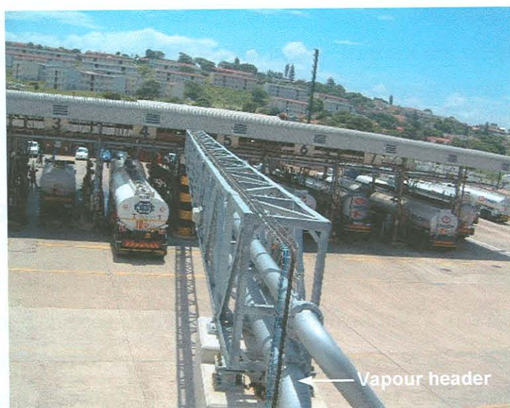
Figure 3.2 Loading racks and vapour header leading to VRU.
