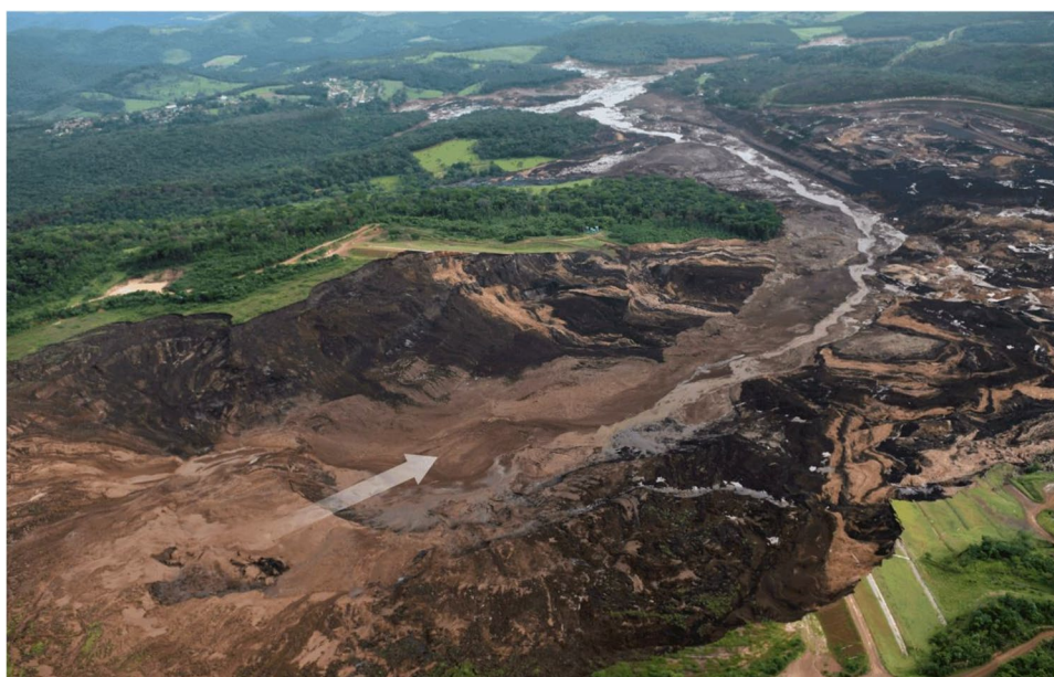
Fig. 3 Collapse of the Brumadinho dam in Mina Córrego do Feijo [2]
