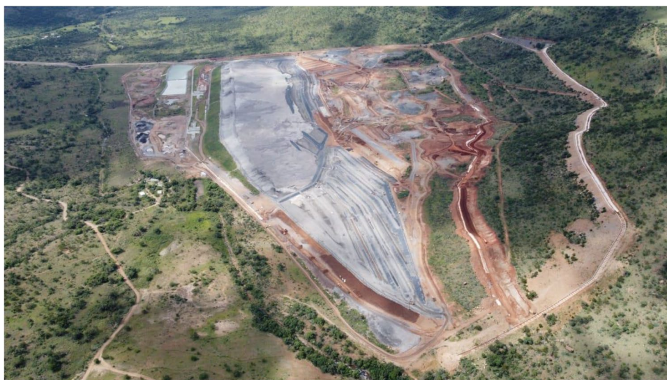
Fig. 16 Mareesburg TFSF ongoing construction
