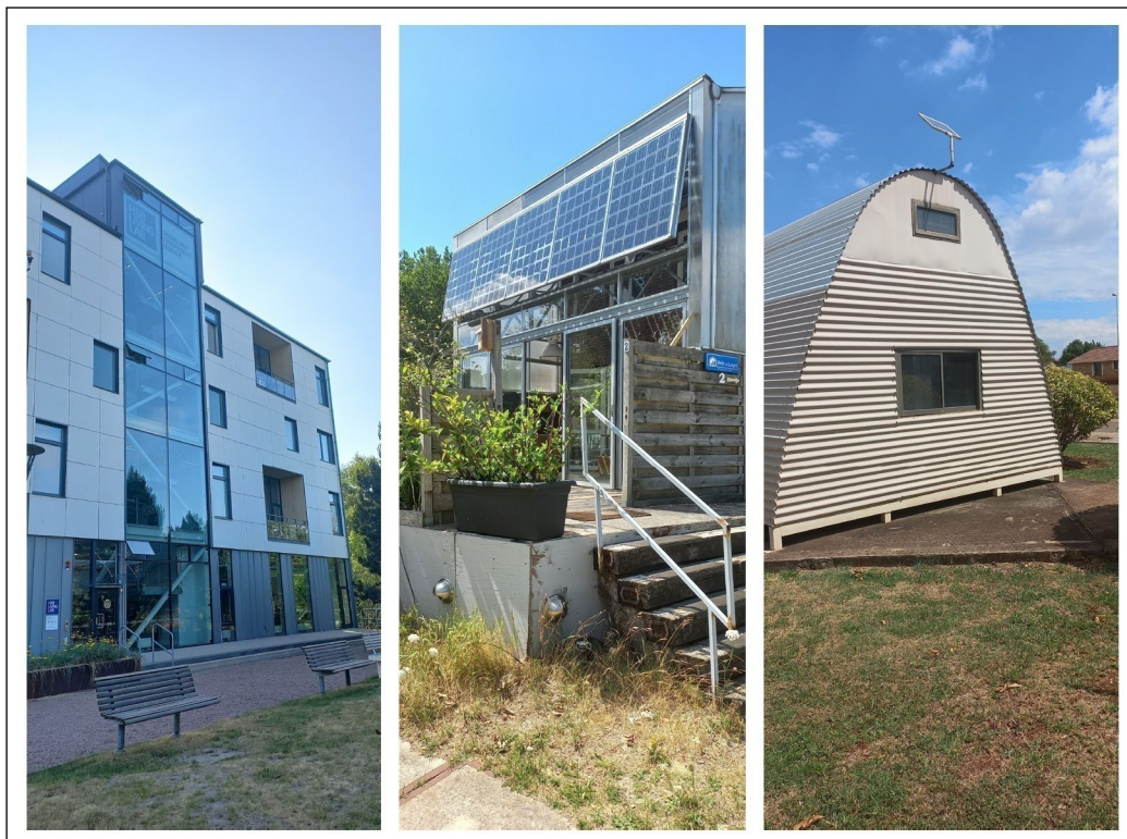
Figure 2: Building technology laboratories (BTLs) and living labs (LLs) reviewed as case studies in Sweden, the Netherlands and South Africa.
