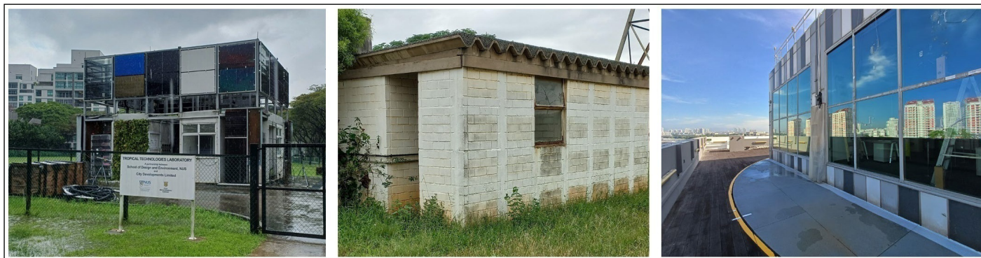
Figure 1: Building technology laboratories (BTLs) reviewed as case studies in Singapore and South Africa.
