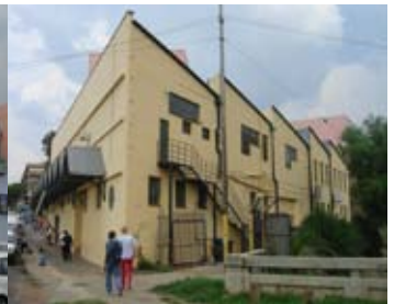
FIGURE 33 (bottom second from left) NAME: Sterland. FEATURES: Sterland movie complex and Hotel. SIGNIFICANCE: Sterland is one of the few remaining movie and entertainment buildings located outside a mall complex.
