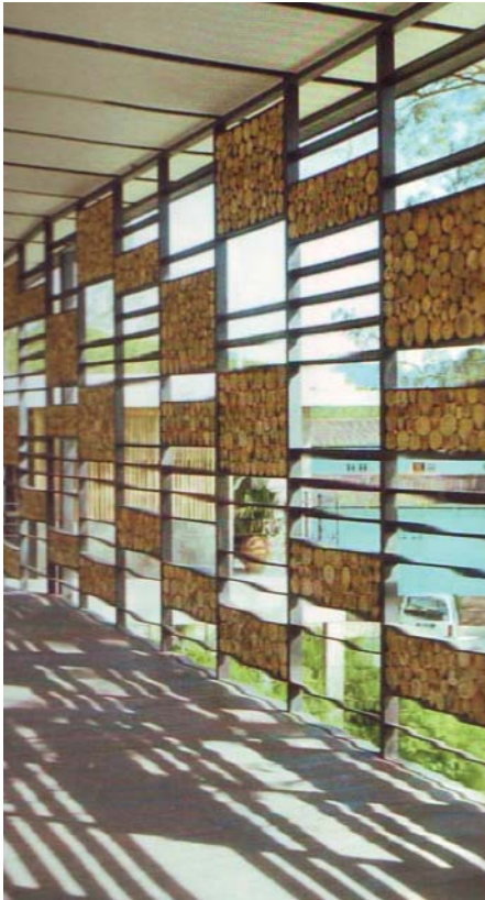
20. BOH Visitors Centre - Metalwork & Timber Screen
