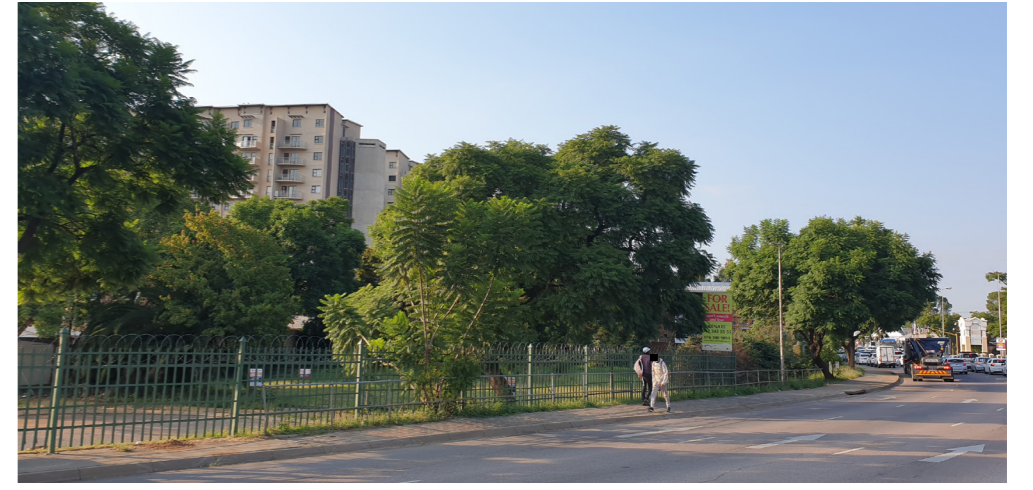
Pedestrians moving past and through dilapidated spaces
