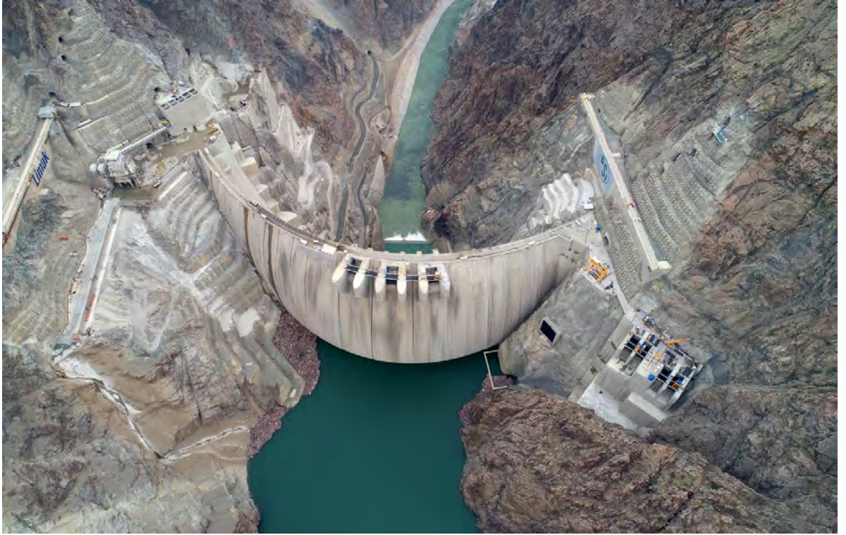
Figure 10-17: Yusufeli Dam reservoir elevation 610 mASL, 137 days after commencement of impoundment (8 April 2023)
