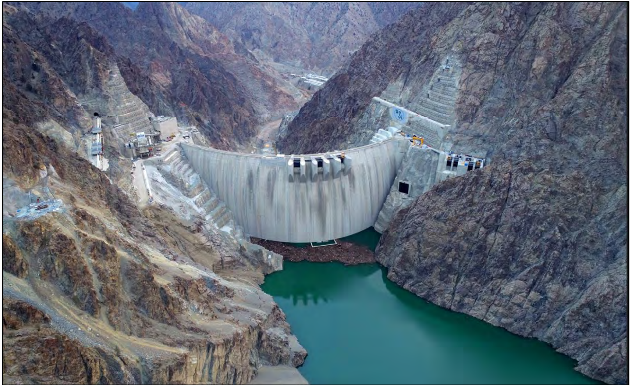
Figure 10-11: Yusufeli Dam reservoir elevation 561.5 mASL, 41 days after commencement of impoundment (2 January 2023)
