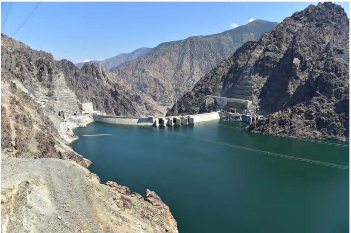
Figure 10-22: Yusufeli Dam reservoir elevation 696 mASL, 269 days after commencement of impoundment (18 August 2023)
