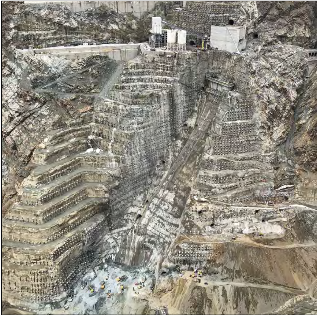
Figure 3-10: Advanced stage of excavation on the left abutment
