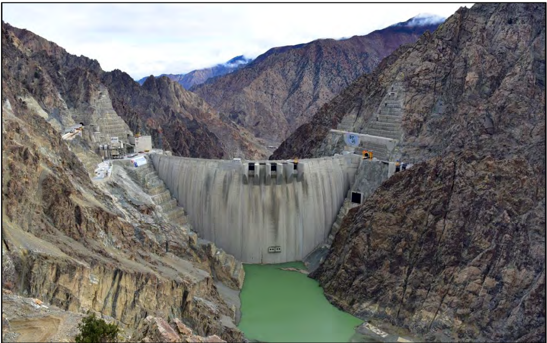
Figure 10-8: Yusufeli Dam reservoir elevation 529 mASL, 4 days after commencement of impoundment (26 November 2022)
