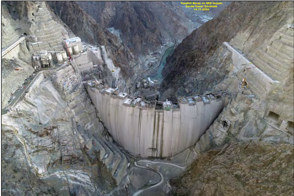
Figure 3-23: Advanced stage of construction showing upstream face of dam
