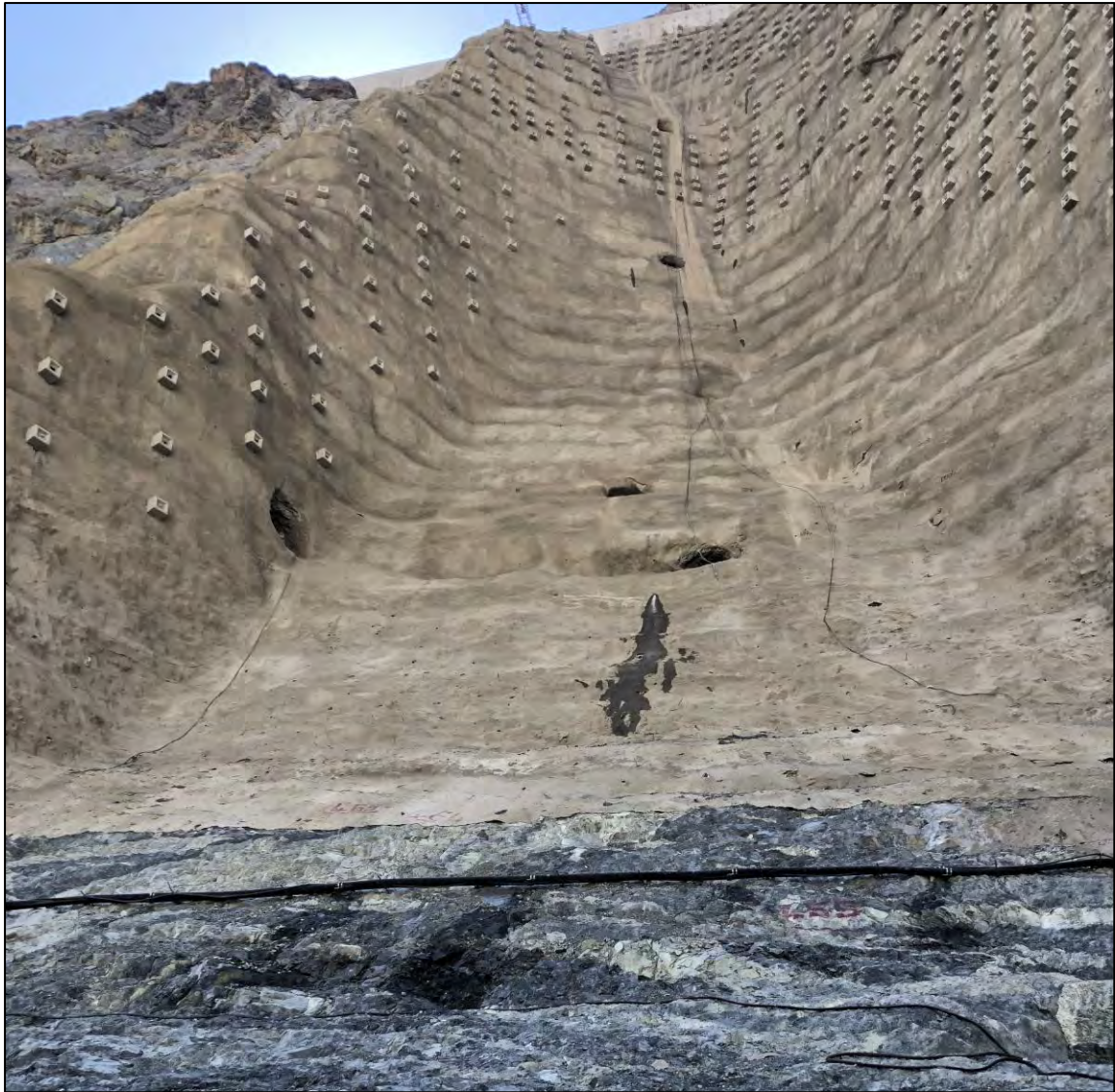
Figure 3-11: Steep excavation surface on right abutment, protected with shotcrete
