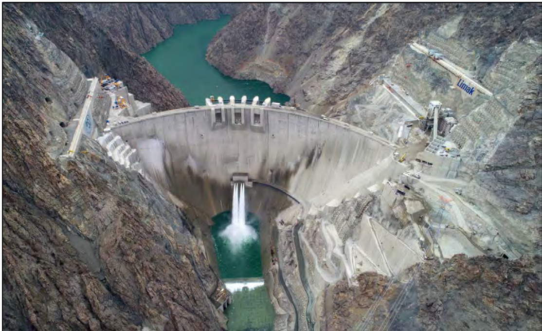
Figure 3-1: Yusufeli Dam reservoir flow release through outlet during impoundment
