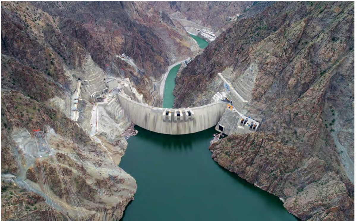
Figure 10-18: Yusufeli Dam reservoir elevation 630 mASL, 159 days after commencement of impoundment (30 April 2023)
