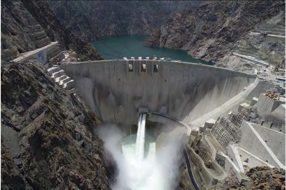
Figure 10-21: Yusufeli Dam reservoir elevation 670 mASL, 200 days after commencement of impoundment (10 June 2023)
