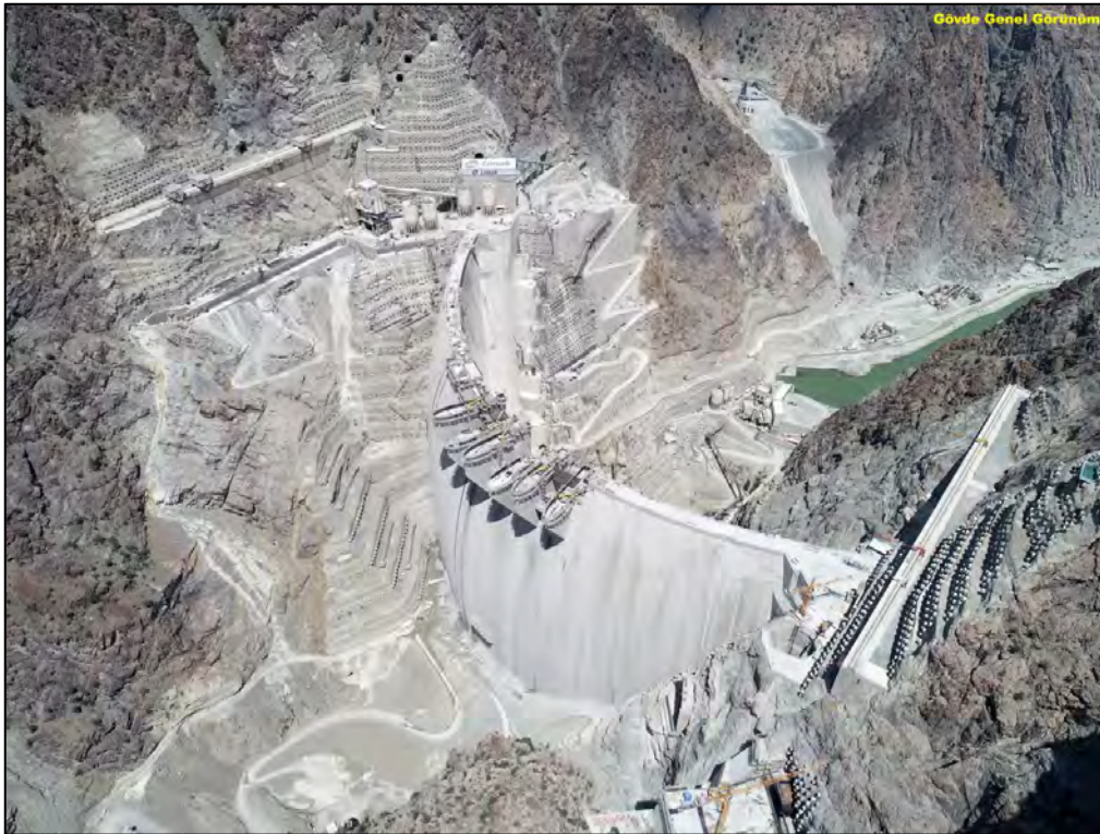
Figure 3-24: Final stages of concrete construction of Yusufeli Dam
