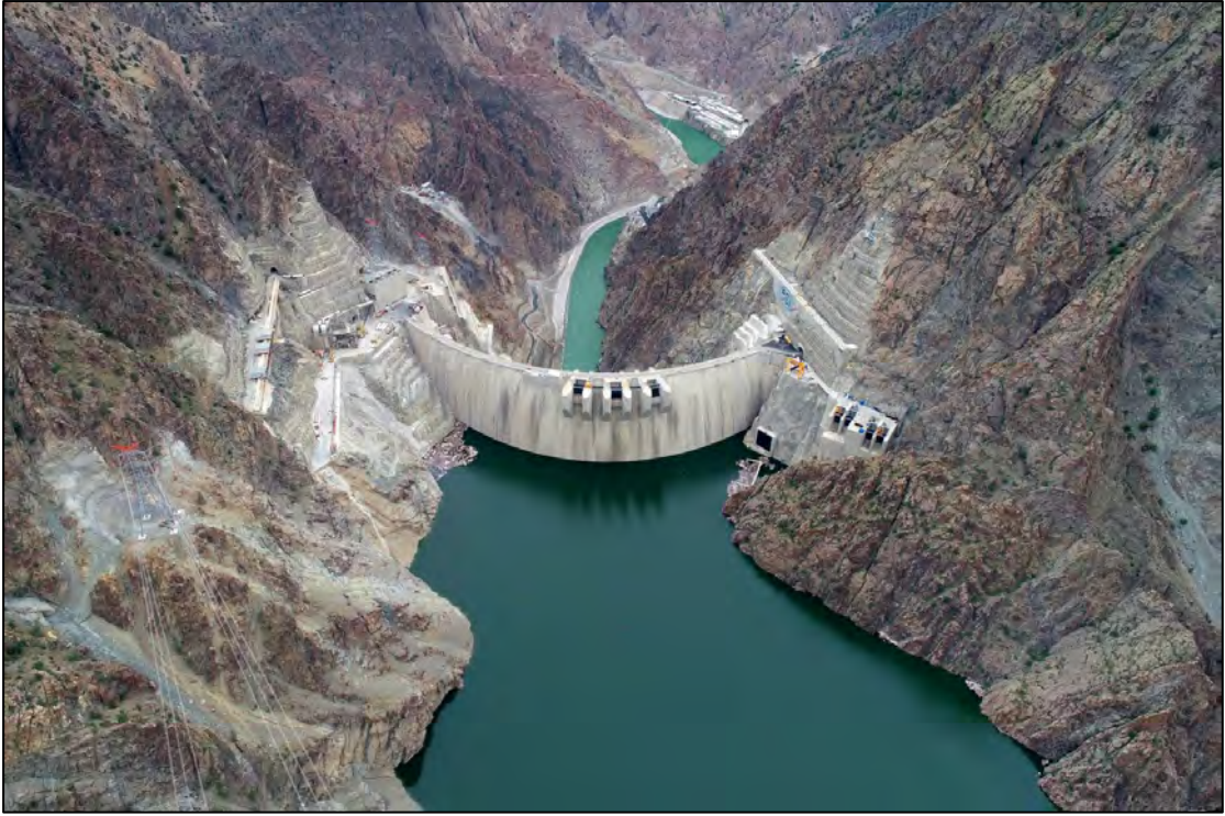
Figure 3-28: Yusufeli Dam reservoir impoundment level 630 mASL (190 m above foundation)
