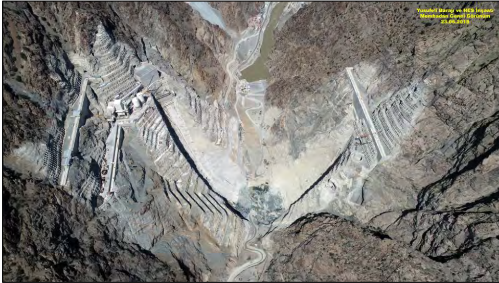
Figure 3-14: View of foundation excavation looking in the direction of stream flow
