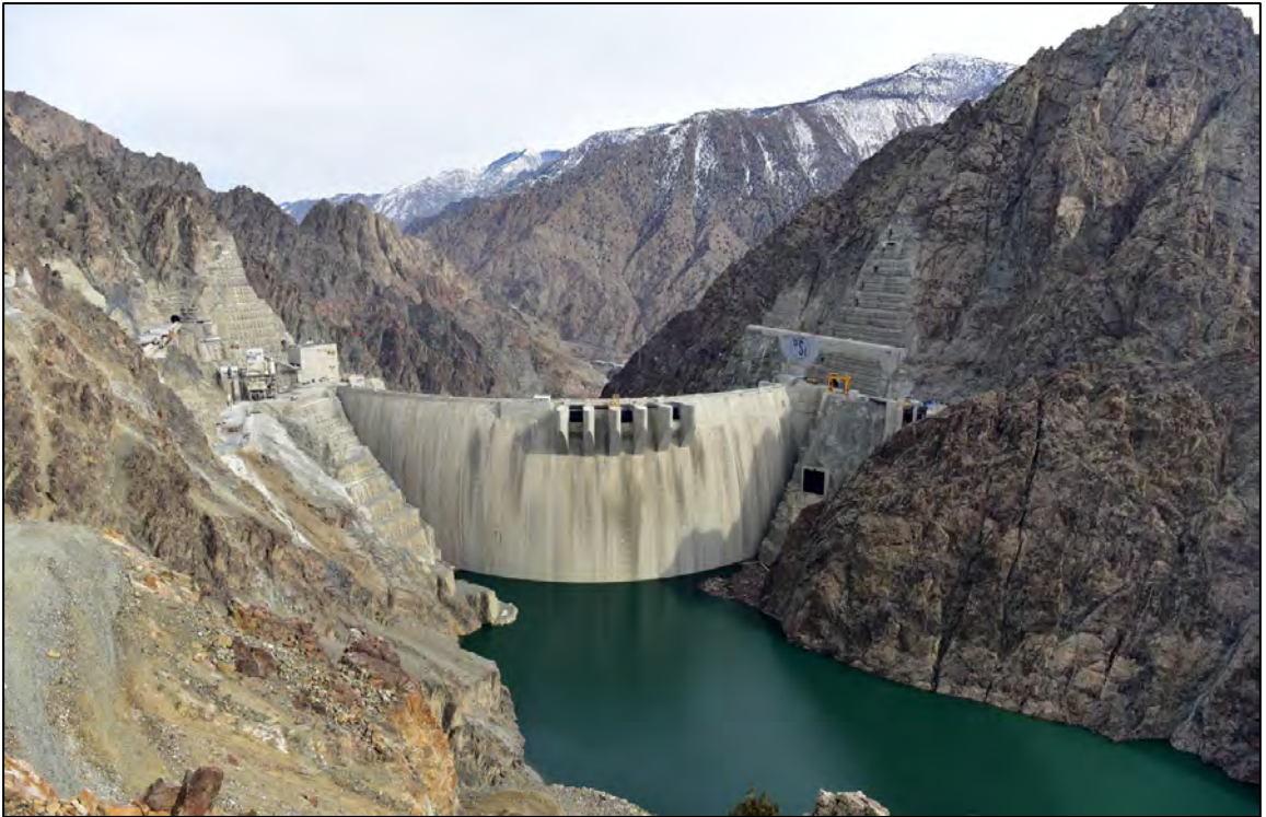
Figure 10-13: Yusufeli Dam reservoir elevation 577 mASL, 74 days after commencement of impoundment (4 February 2023)
