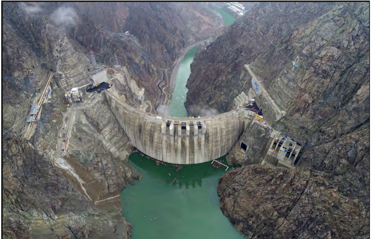
Figure 10-16: Yusufeli Dam reservoir elevation 588 mASL, 124 days after commencement of impoundment (26 March 2023)
