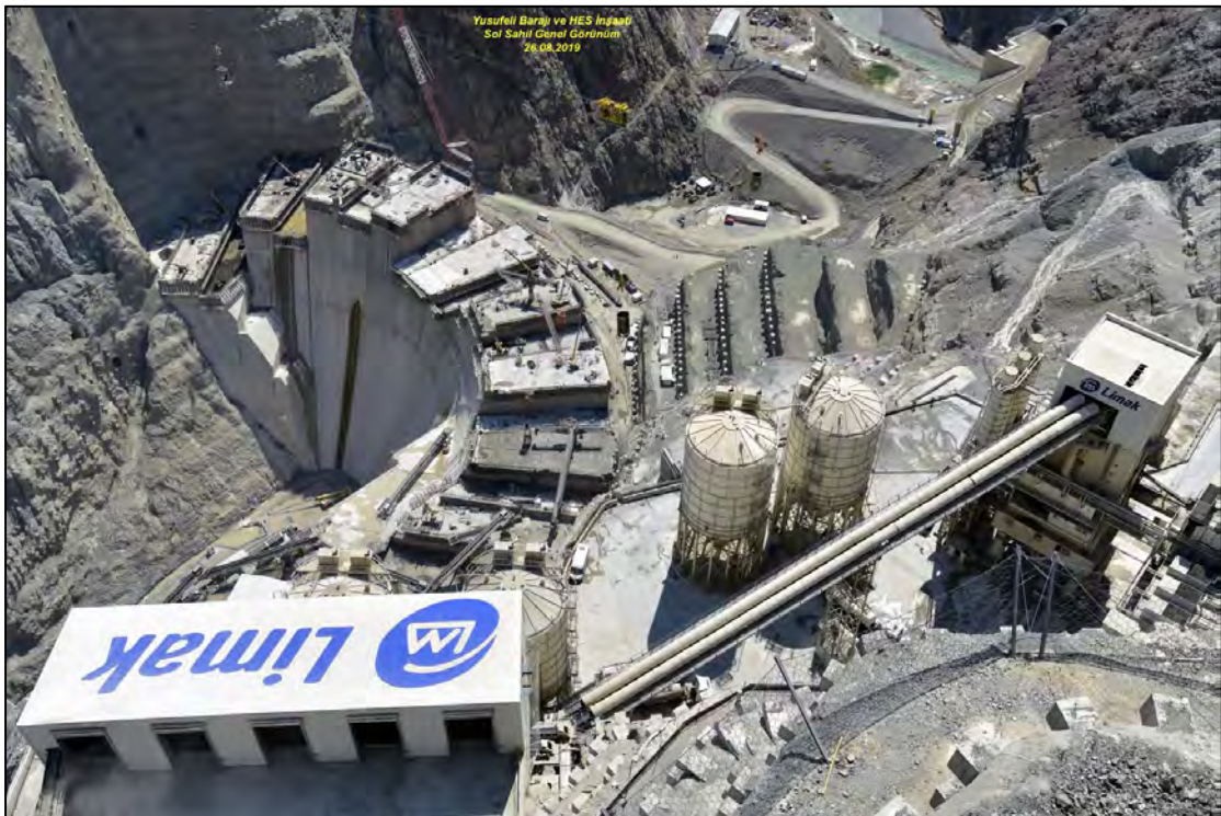
Figure 3-16: Concrete batch plant and cooling plant on upper left abutment
