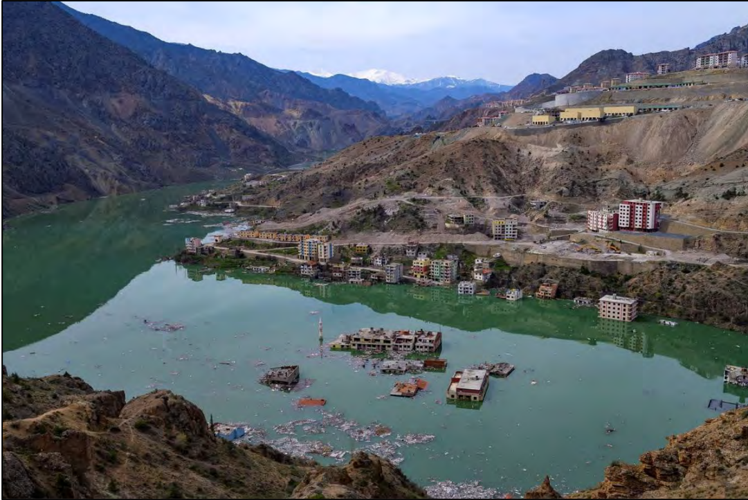
Figure 3-33: Inundation of Yusufeli town upstream of dam on the banks of the Coruh River
