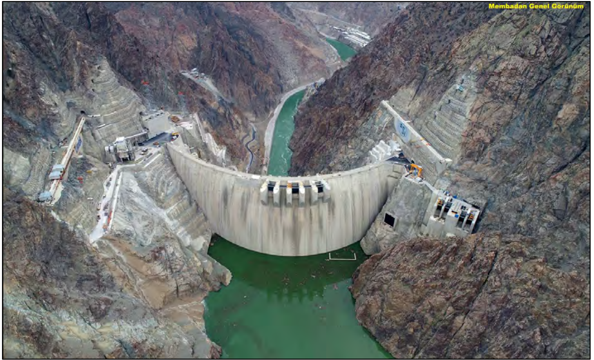
Figure 10-15: Yusufeli Dam reservoir elevation 582 mASL, 117 days after commencement of impoundment (19 March 2023)
