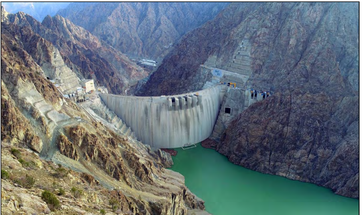
Figure 10-10: Yusufeli Dam reservoir elevation 550 mASL, 22 days after commencement of impoundment (14 December 2022)
