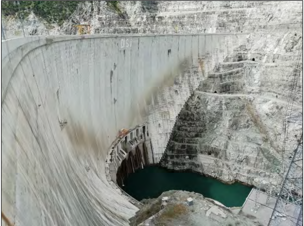
Figure 3-3: General photograph of the downstream face of Deriner Arch Dam
