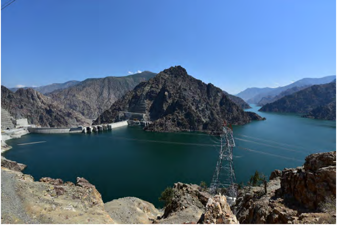
Figure 10-23: Yusufeli Dam reservoir elevation 696 mASL, 269 days after commencement of impoundment (18 August 2023)
