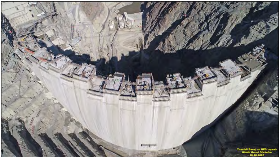
Figure 3-22: Casting of concrete monoliths using leader-follower block approach
