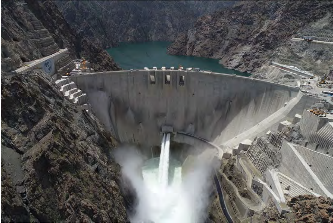
Figure 3-32: Downstream view of Yusufeli Dam reservoir impoundment to level 230 m above foundation
