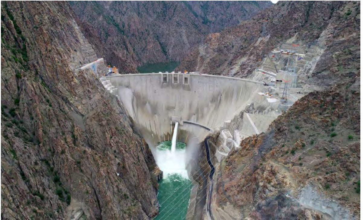
Figure 10-19: Yusufeli Dam reservoir elevation 630 mASL, 159 days after commencement of impoundment (30 April 2023)
