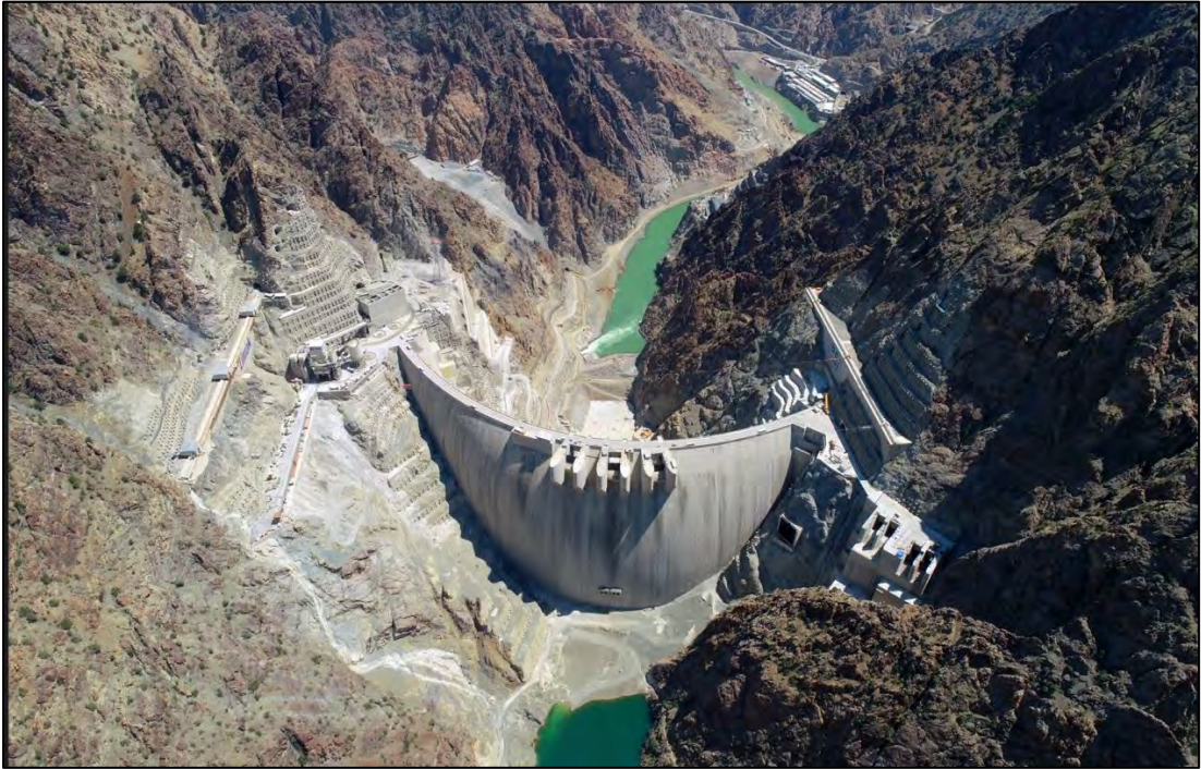
Figure 10-7: Yusufeli Dam reservoir elevation 503 mASL, shortly before commencement of reservoir impoundment (15 November 2022)
