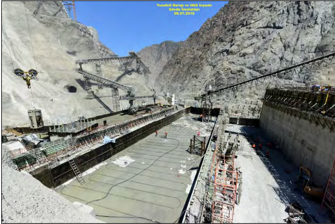
Figure 3-19: Delivery of concrete with conveyor belts from upstream & downstream and bucket
