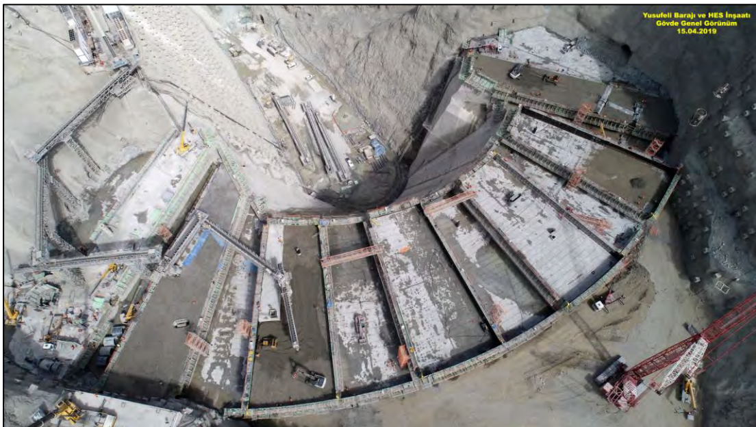
Figure 3-20: Early stages of concrete placement in dam body
