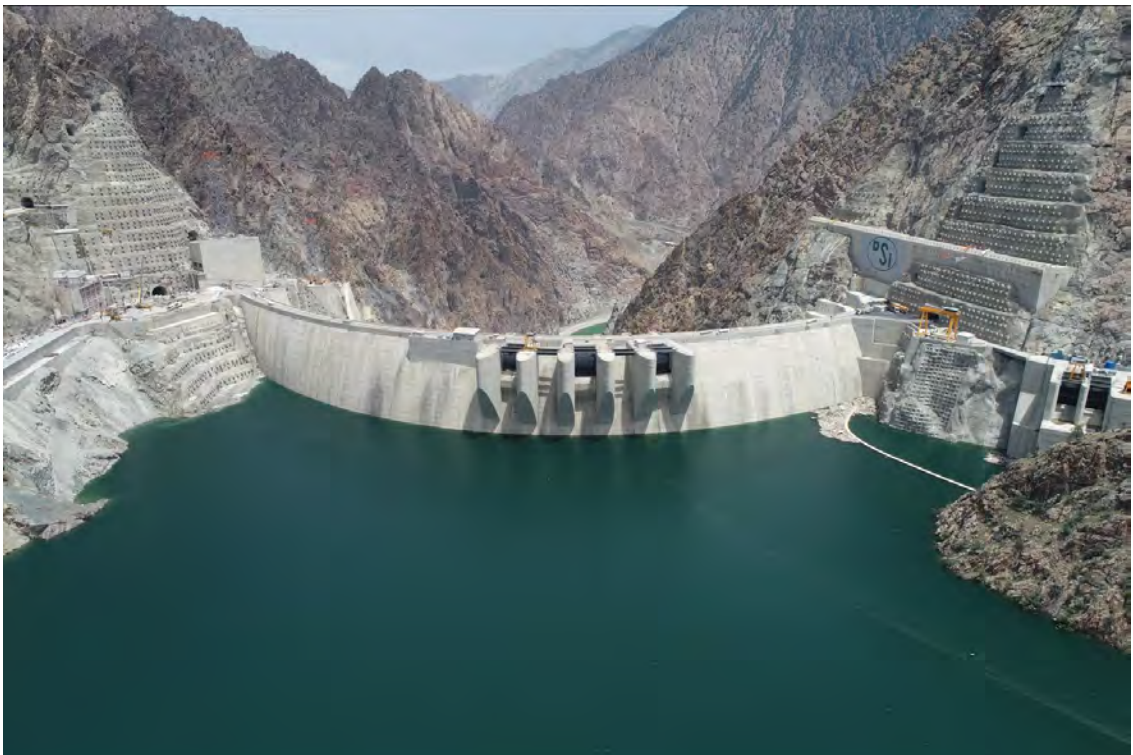
Figure 3-29: Yusufeli Dam reservoir impoundment level 670 mASL (230 m above foundation)
