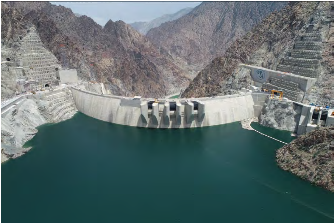
Figure 10-20: Yusufeli Dam reservoir elevation 670 mASL, 200 days after commencement of impoundment (10 June 2023)
