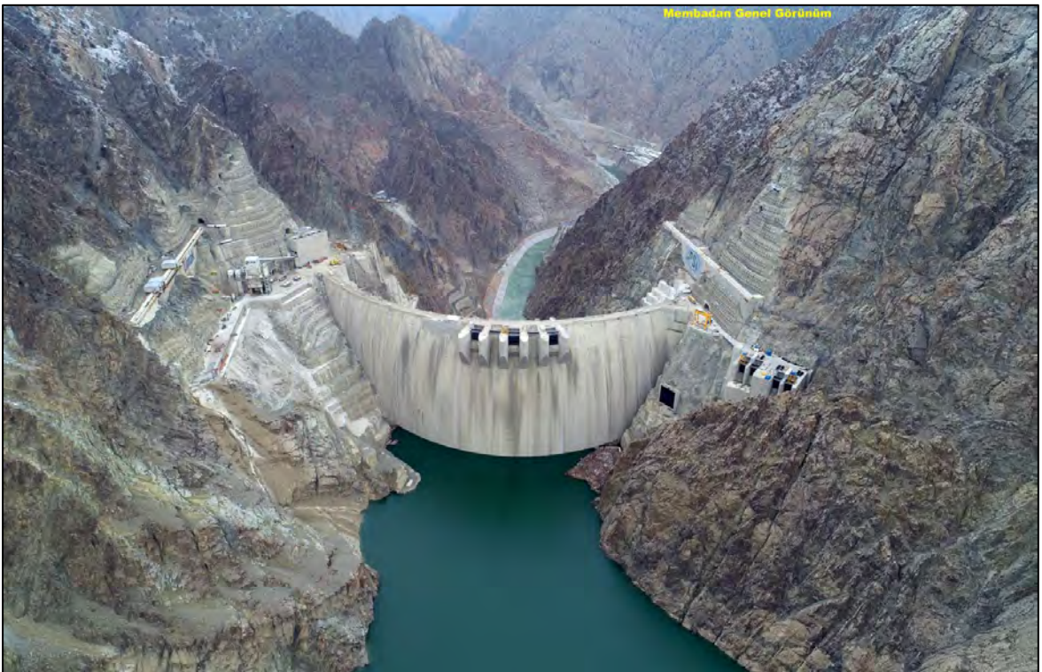
Figure 10-14: Yusufeli Dam reservoir elevation 580 mASL, 96 days after commencement of impoundment (26 February 2023)
