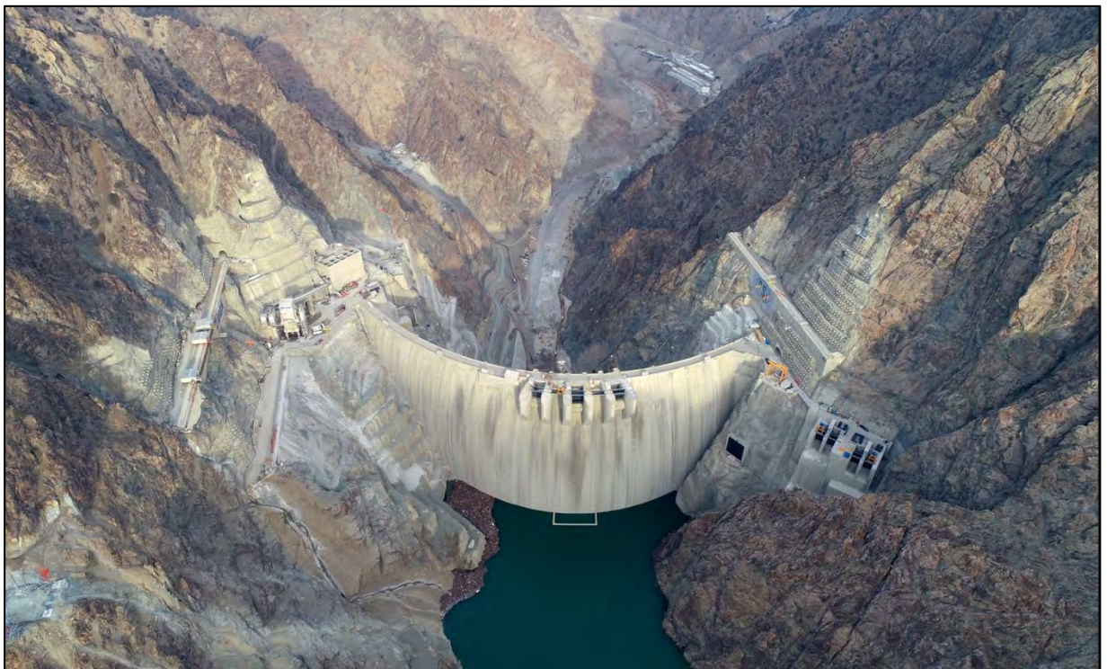
Figure 10-12: Yusufeli Dam reservoir elevation 574 mASL, 63 days after commencement of impoundment (24 January 2023)
