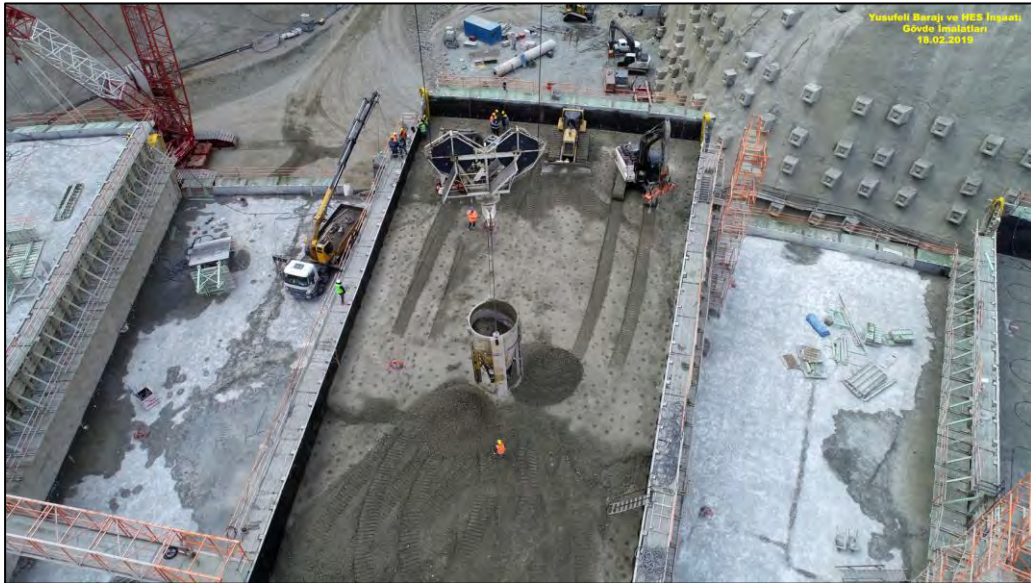
Figure 3-17: Placement of concrete with 9 m 3 bucket suspended from cable crane
