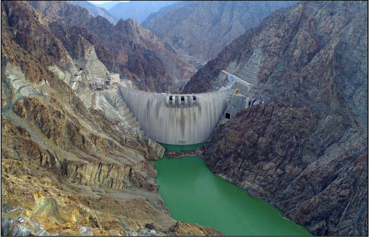
Figure 10-9: Yusufeli Dam reservoir elevation 536 mASL, 8 days after commencement of impoundment (30 November 2022)
