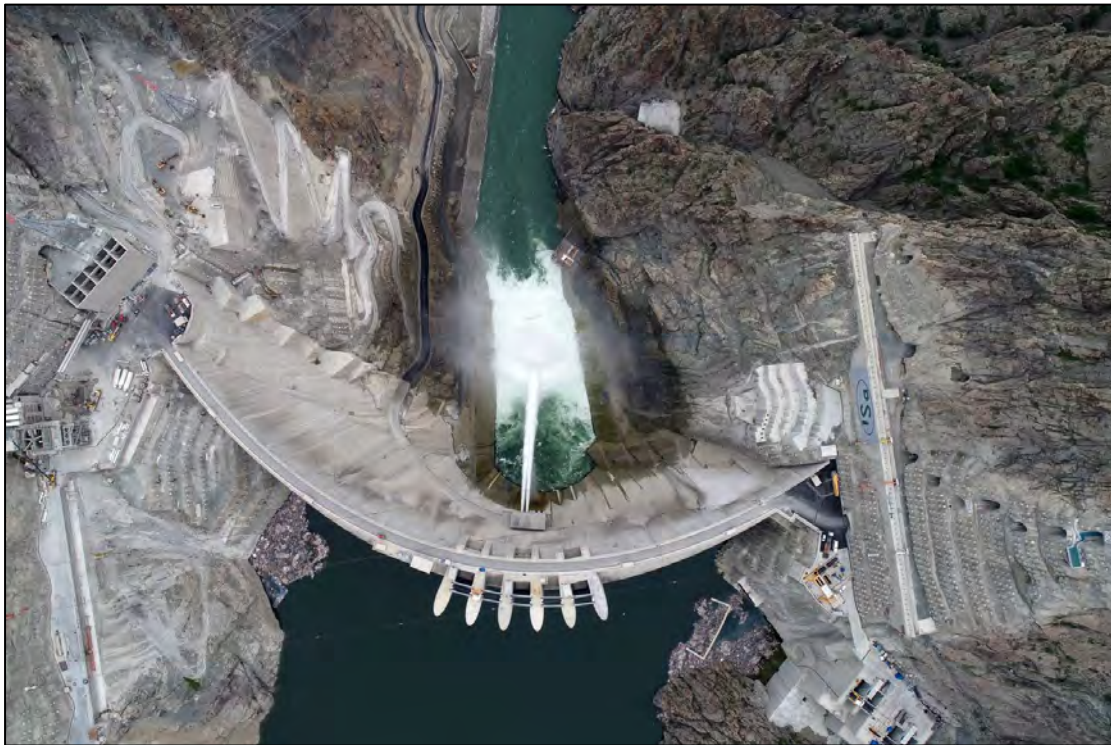
Figure 3-31: Aerial view of Yusufeli Dam reservoir impoundment to level 200 m above foundation
