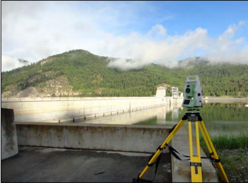
Figure 2-55: Total station with EDM capability set up for measuring dam movements (USACE, 2018)
