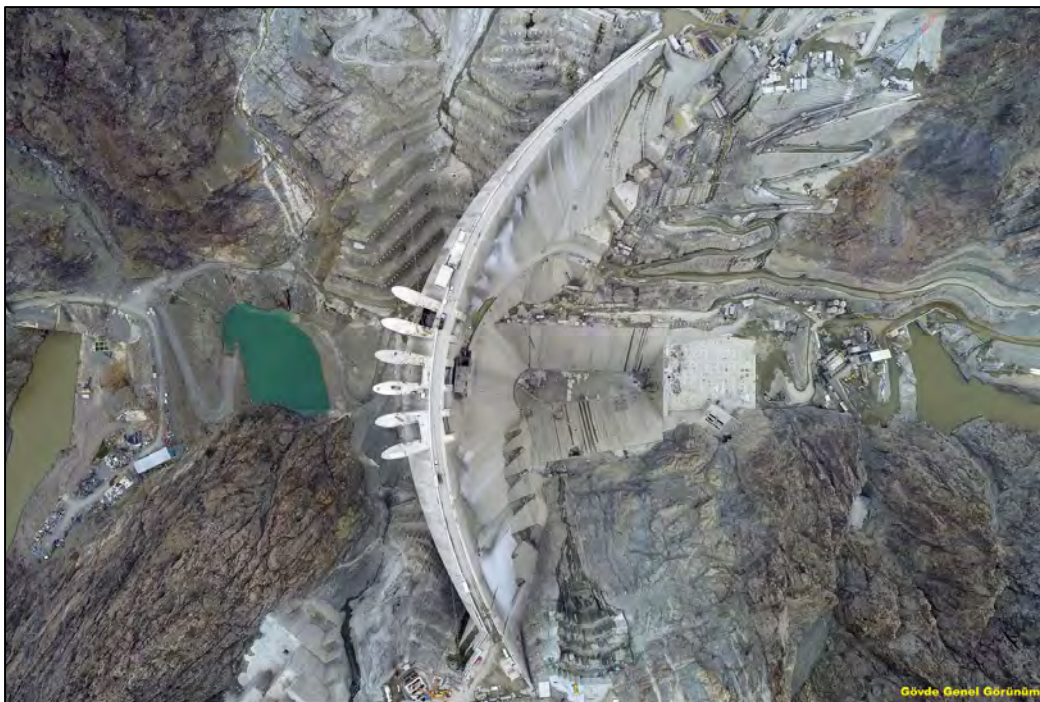
Figure 3-27: Aerial view of the completed Yusufeli Dam orientated with upstream on the left
