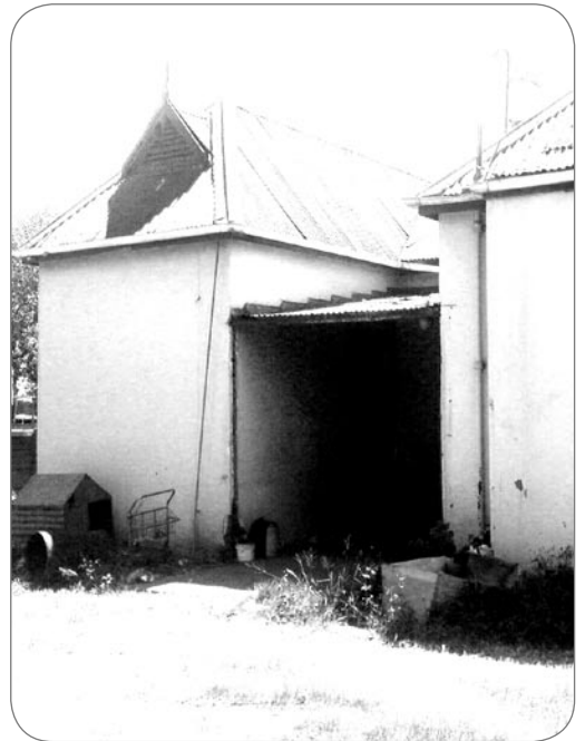
fig. 8.6 rear view of building
