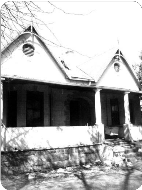
fig. 8.5 front view of building
