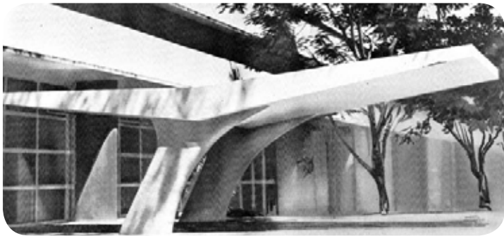
fig. 6.5 column investigation_sketch 6.6 school entrance canopy, Brazil_Oscar Niemeyer 6.7 concept sketch_columns 6.8 t-frame structure 6.9 Perspective view of roof form
