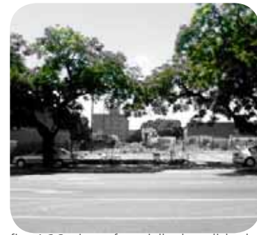
fig. 4.26 view of partially-demolished site, 28 February 2007
