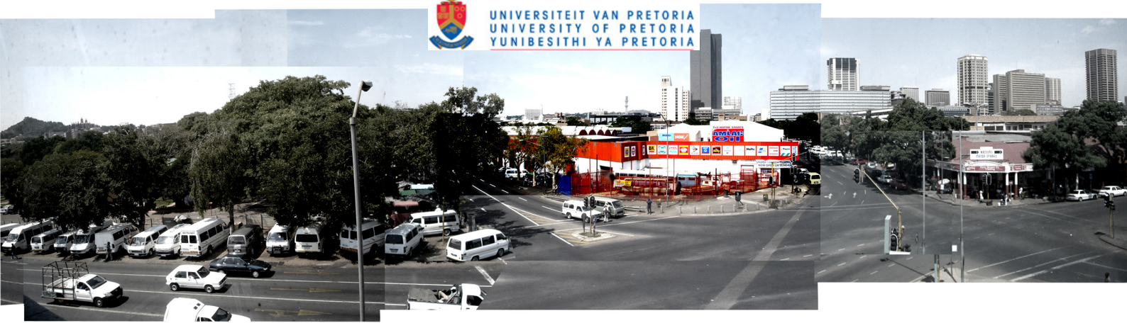
Fig. 1.23 Panoramic view of the site and the intersection. This image explains the visual importance the site already has through the display of large merchandise boards on the corner of the existing building
