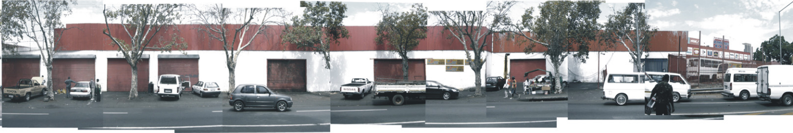
Fig. 1.27 Elevation of Du Toit street showing the state of the buildings and activities happening in the street.
