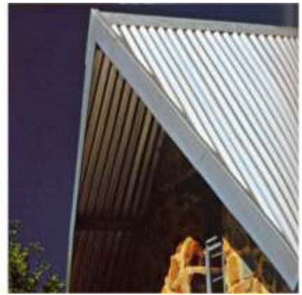
Figure 7.54: Contemporary fascia detail for steel roofs
