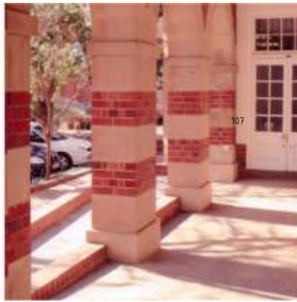
Figure 7.53: Typical sandstone and brick (english bond) construction
