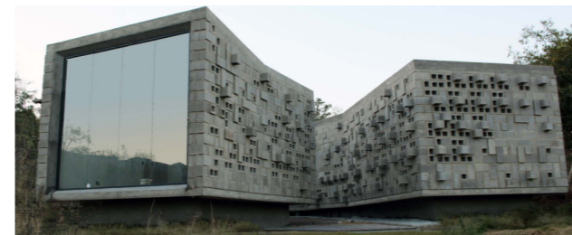
Seed bank: Local used concrete block by Paragon architects
