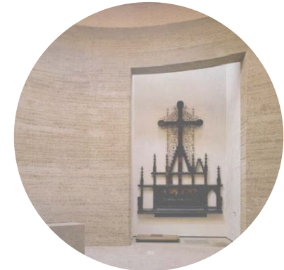
RECESSES WITHIN THE RAMMED EARTH SANCTUARY
