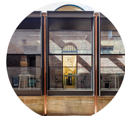
NEW GLASS FACADE STEPS AWAY SIGNIFICANTLY FROM THE OLD FACADE
