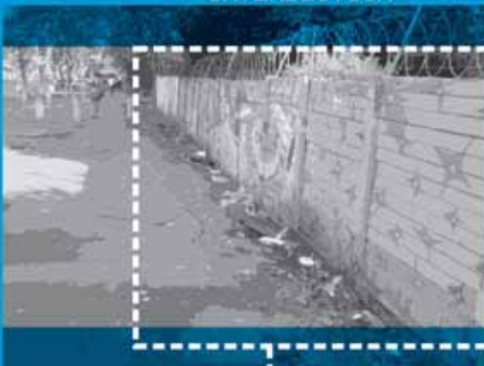
→ PRECAST CONCRETE WALL
