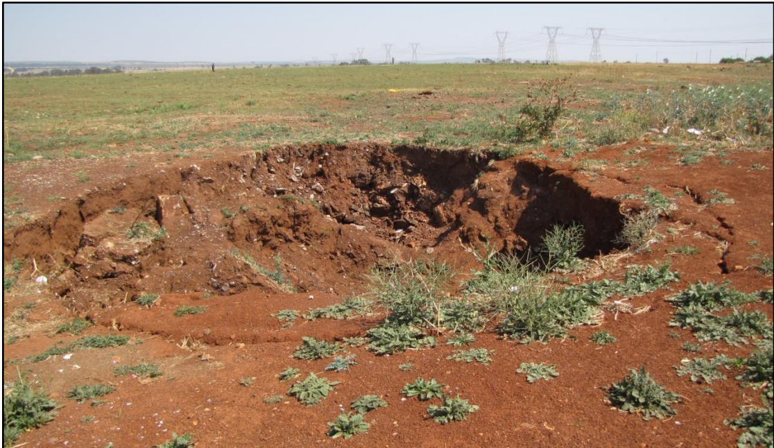
Figure 13: Recent caving of the ground surface forming a subsidence (Photo from CGS Database).
