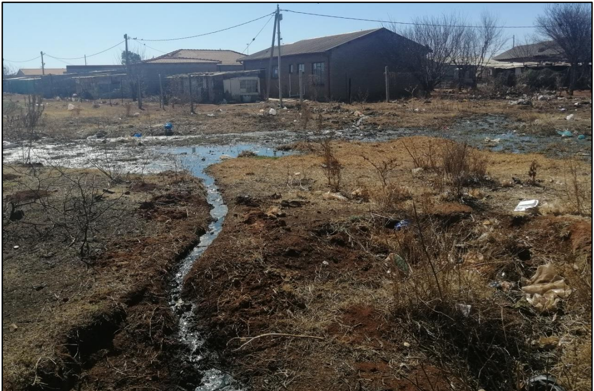
Figure 23: Blocked and back-ponding sewage effluent flowing into open field and sinkholes.
