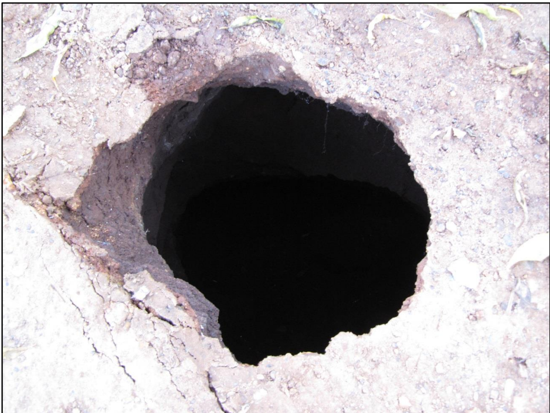
Figure 11: Recently collapsed arch forming a small sinkhole (Photo from CGS Database).
