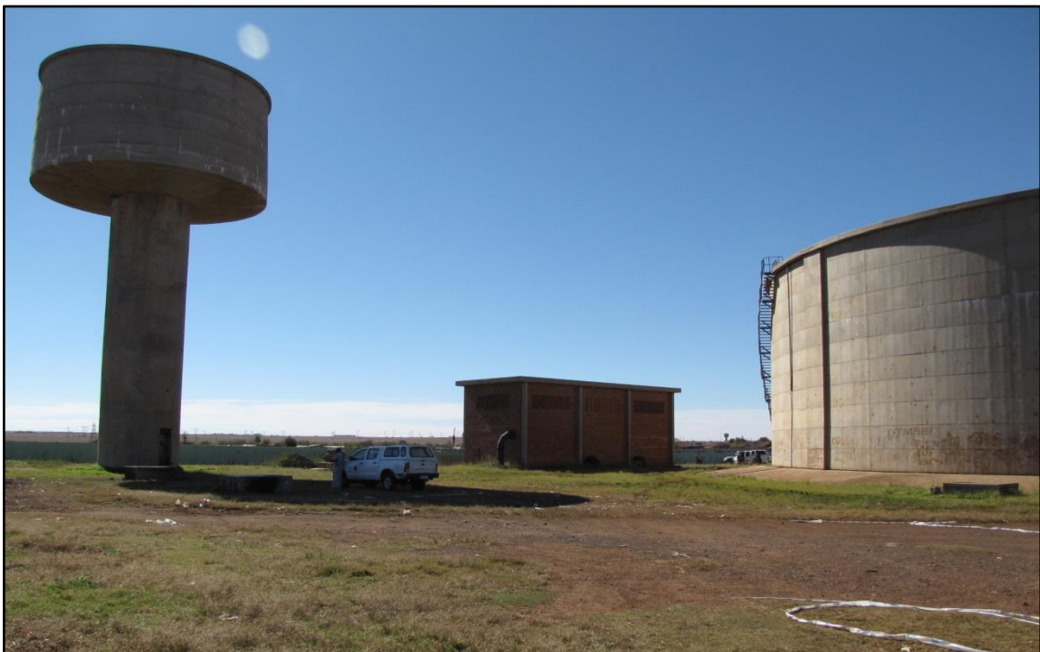
Figure 44: A decommissioned Khutsong Main Reservoir, border of Khutsong Extension 3 and 6.
