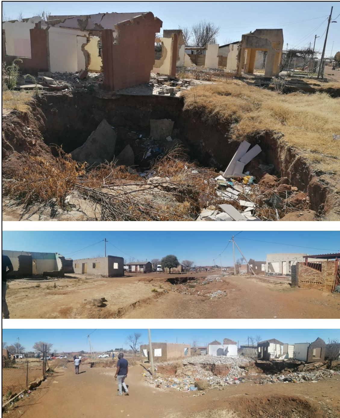
Figure 38: Trail of destruction to housing at Adatite Street, Khutsong Proper.
