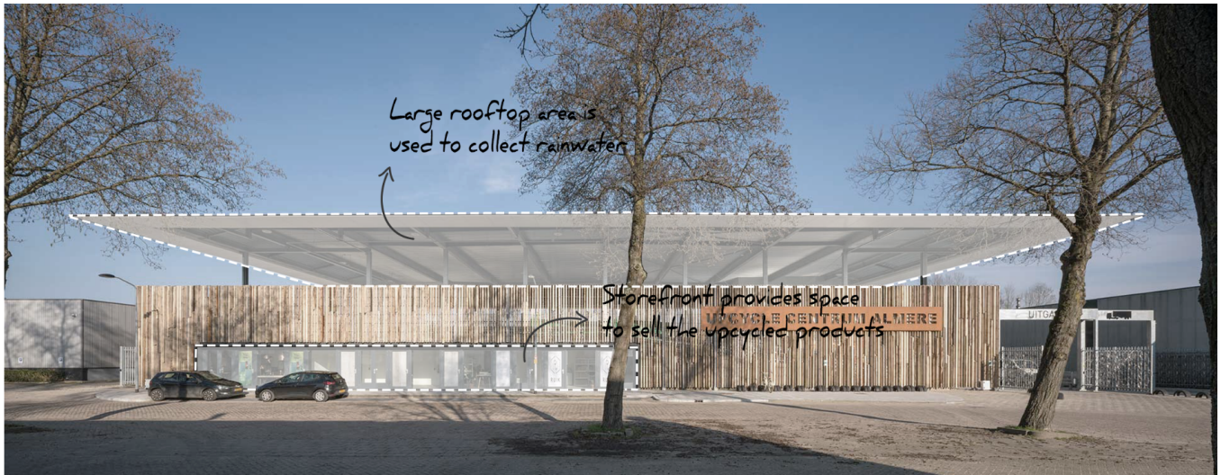
Figure 2.11: The Upcycle-Centrum Almere with rainwater collection roof and a public interface for upcycled products (LKSVD 2018)
