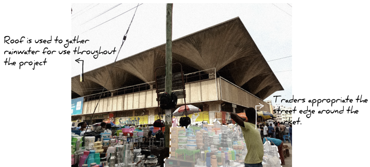
Figure 2.10: Traders appropriate street edge as the informal market has outgrown the existing space
