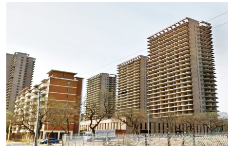
Fig 3.4 Dilapidated Schubart Park (Google Street View 2020)
