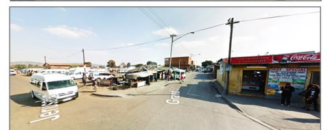
Fig 3.6 Various structures throughout Marabastad showing signs of decay. (Google Street View 2020)
