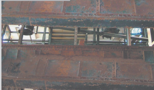
Fig. 7.2_ interior of Retort house, indicating re-use of salvaged materials
