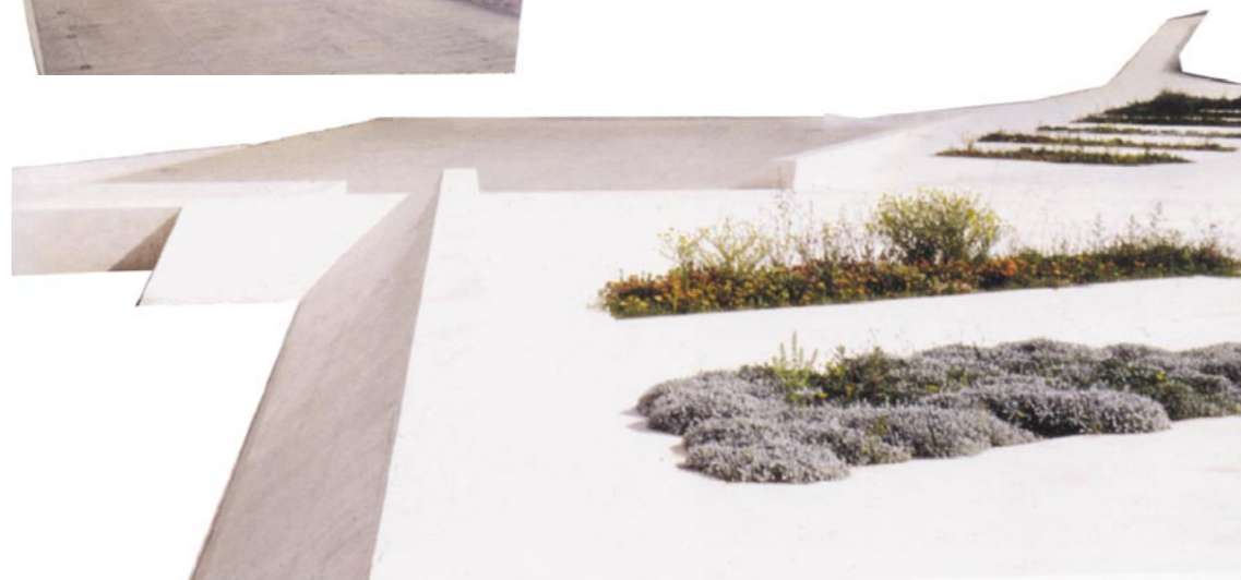
Fig. 117 Planter laid flush in concrete screed. J. Miguel Hernandes León, Murallas de Ceuta, 1992-1999, Ceuta Spanish enclave in Marocco (A. Aymonino, V. P. Mosco 2006: 48)
