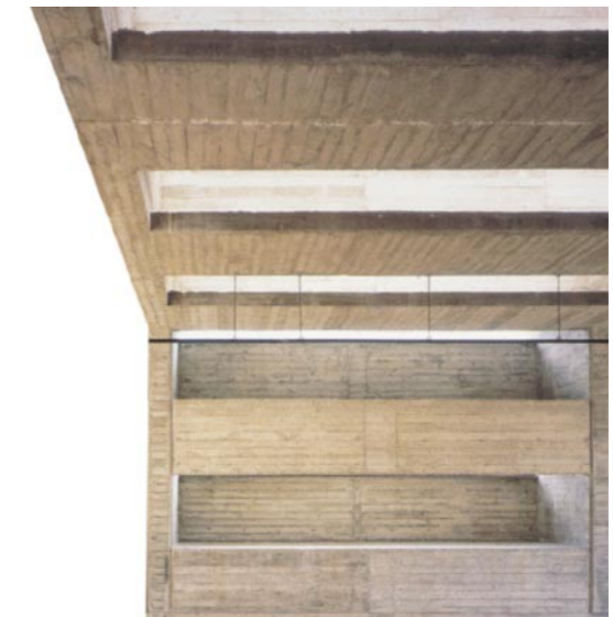
Fig. 113 Off shutter concrete wall patterned by the grain of timber shuttering planks. GPY Architectos. San Bernardo Assembly hall and workshop space, 1999-2001, Los Silos, Tenerife, Spain. (Hadid, Z. Forster, K. Sudjic, D. et al. 2005: 131)
