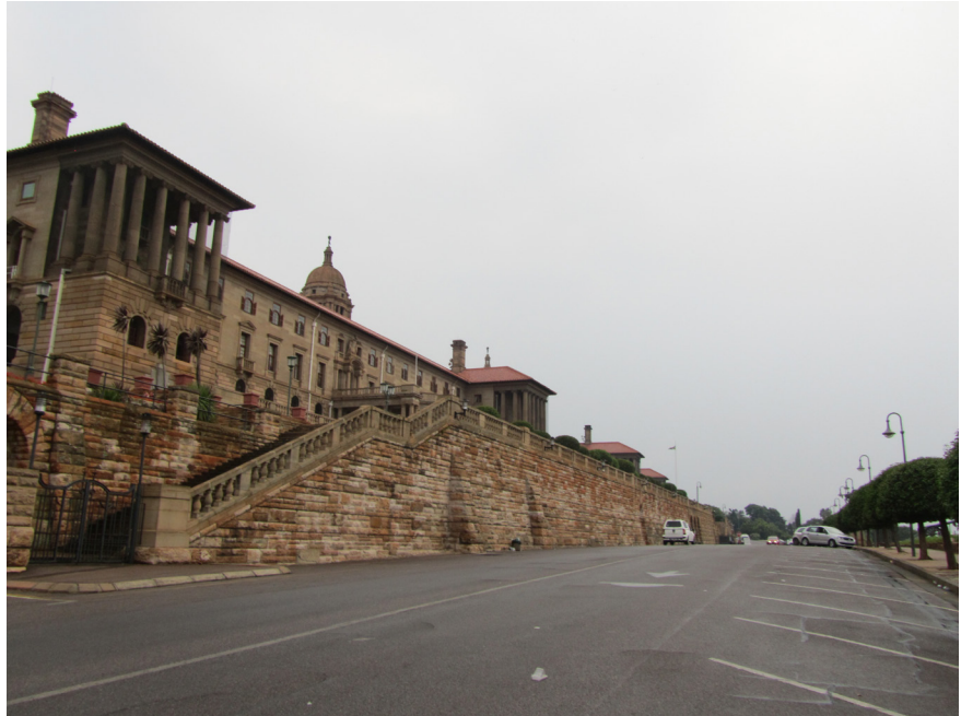
Figure 3.2: Western side view of Union Buildings. The fortified wall further strengthened by a much later addition of the steel fences prohibiting people from entering the second tier road (Author, 2015)
