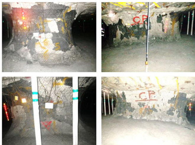
Figure 8—The central instrumented pillar in the pillar project area. This pillar was classified as a Class 3 unstable pillar
