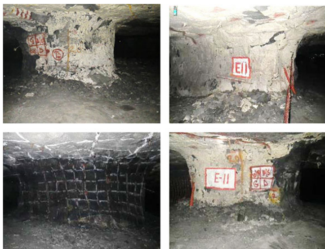
Figure 9—A Class 2 stable pillar in the pillar project area
