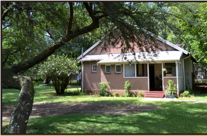
Another of the old Onderstepoort staff houses built c. 1924 where female students lodged from the 1940s to the 1970s, is now rented by the University of Pretoria for student accommodation.
