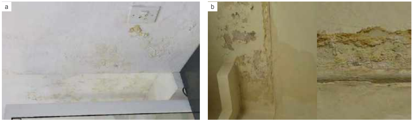
Figure 1: Photographs of visible mould on wall surfaces of areas investigated: (a) clinic room wall with mould growth and (b) X-ray file data storage room.
