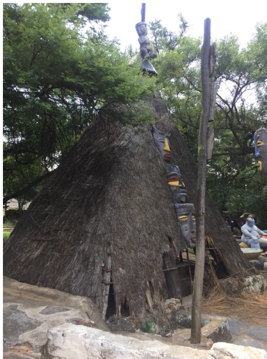
Figure 5.25: Pyramid-shaped indumba at Credo Mutwa's homestead in Soweto. The structure was built with gum poles and thatch (Source: author, 2020)
