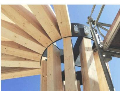
Canopy Structural Components - Heavy-duty connector for mass timber construction up to 768 kN for vertical and ooverhead components
