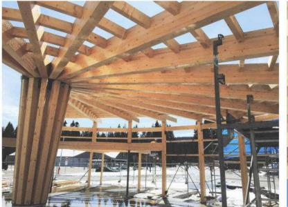
Structure of canopy with the use of Glue Laminated Timber (Glulum) as a material
