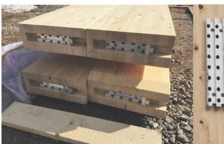
Galvanized Steel connectors for connection of Glulum bracing components
