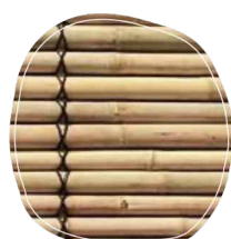
bamboo pole mat (suspended on metal frames below polycarbonate roof)
