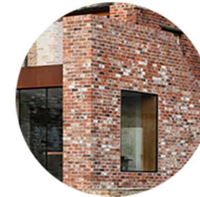
2// SKIN masonry recycled brick infill walls steel windows and doors
