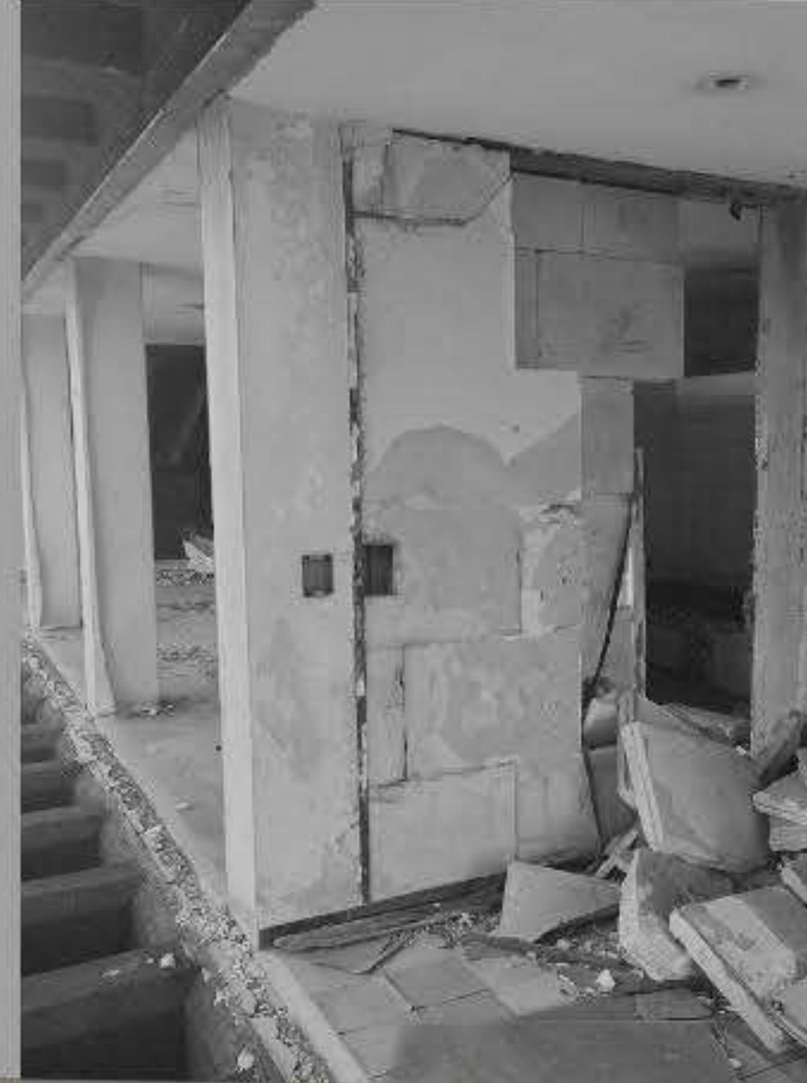
Infill walls to be demolished
