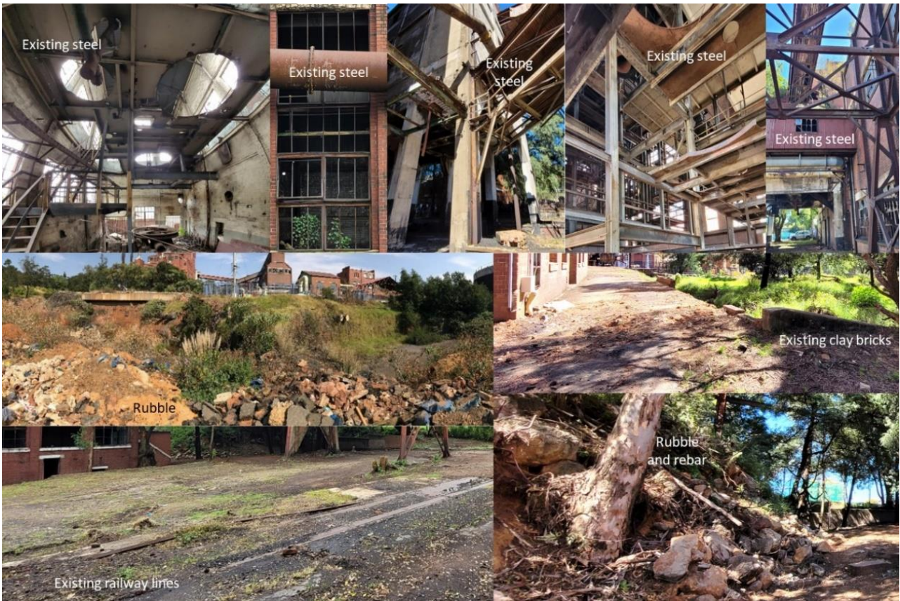
Figure 15: Existing site materials currently present on site.
