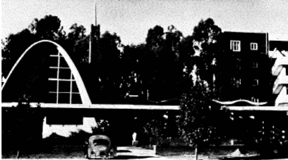
Figure 4 Photocopied Photograph circa 1973 showing the South façade (source: : Cummins 1973: 8, unknown photographer).
