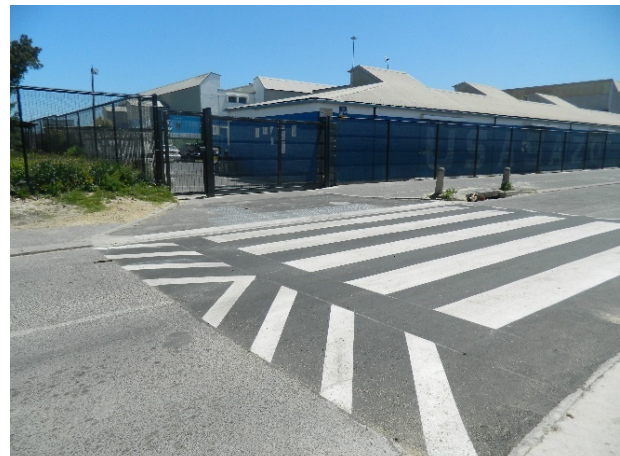
Modified Usasazo High school entrance
