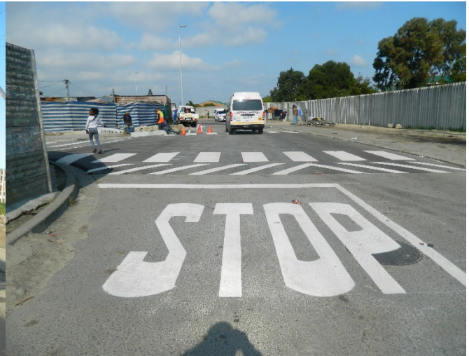
Raised Intersection of Bangiso Drive and Lelala Crescent after modifications
