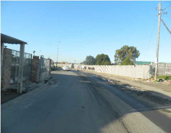
Intersection of Bangiso Drive and Lelala Crescent before modifications
