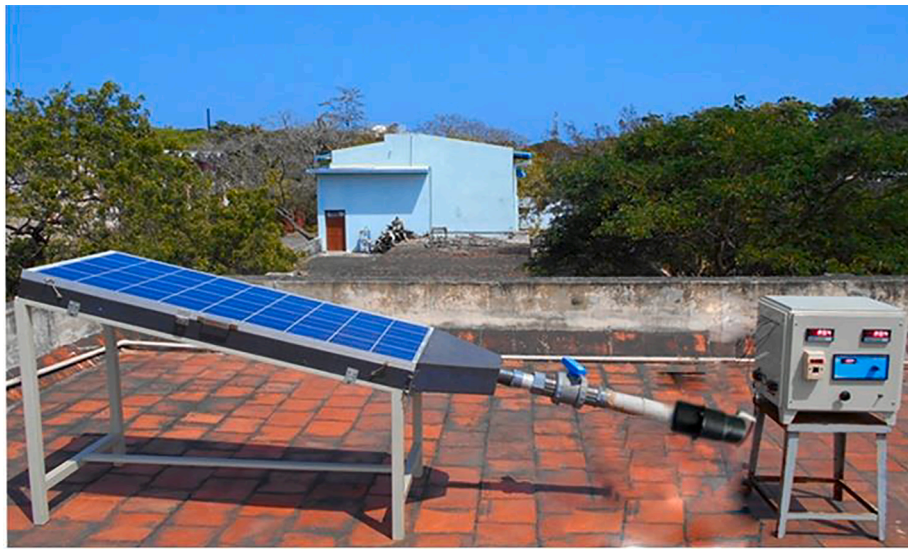
Fig. 1b. Photographic view of PV/T system.
