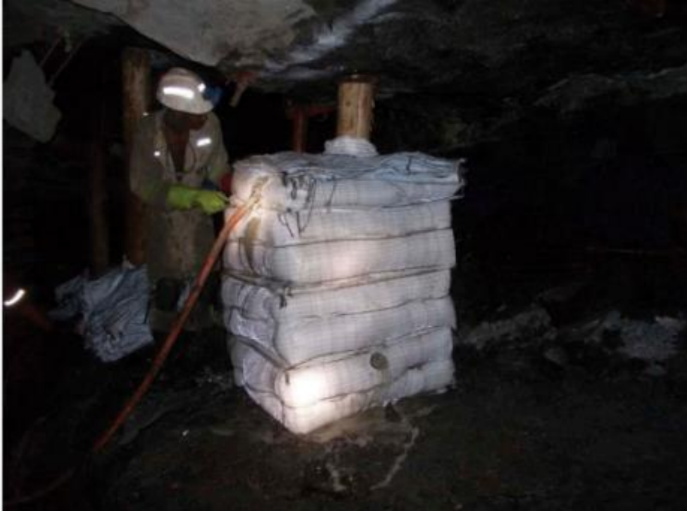
Figure 2-38. Square grout packs (after Van der Spuy, 2021).
