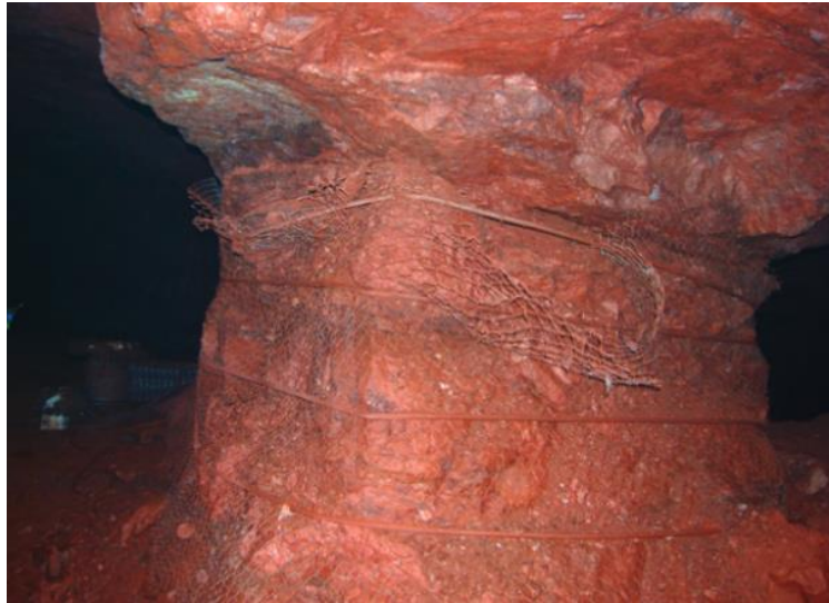
Figure 2-17. Pillar strapping at the Santa Rosa Mine (after Alejano et al., 2017).
