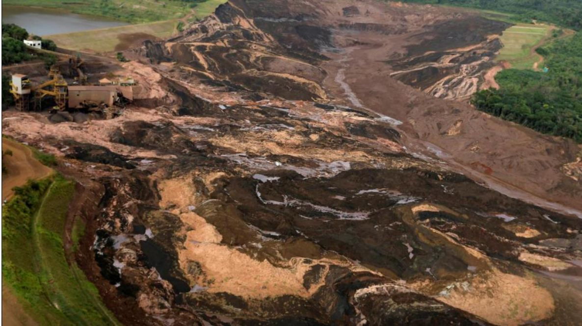
Figure 2-4. The mine cafeteria destroyed by the dam failure (after Boadle and Nogueira, 2019).
