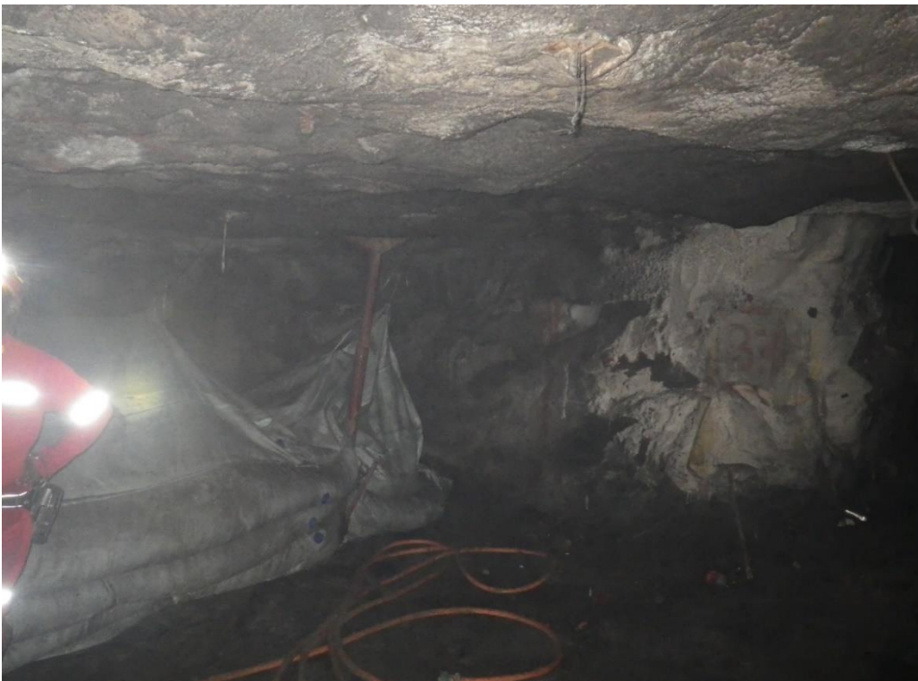
Figure 5-15. Use of backfill bags in an attempt to seal the holing between adjacent pillars (courtesy of D. F. Malan).
