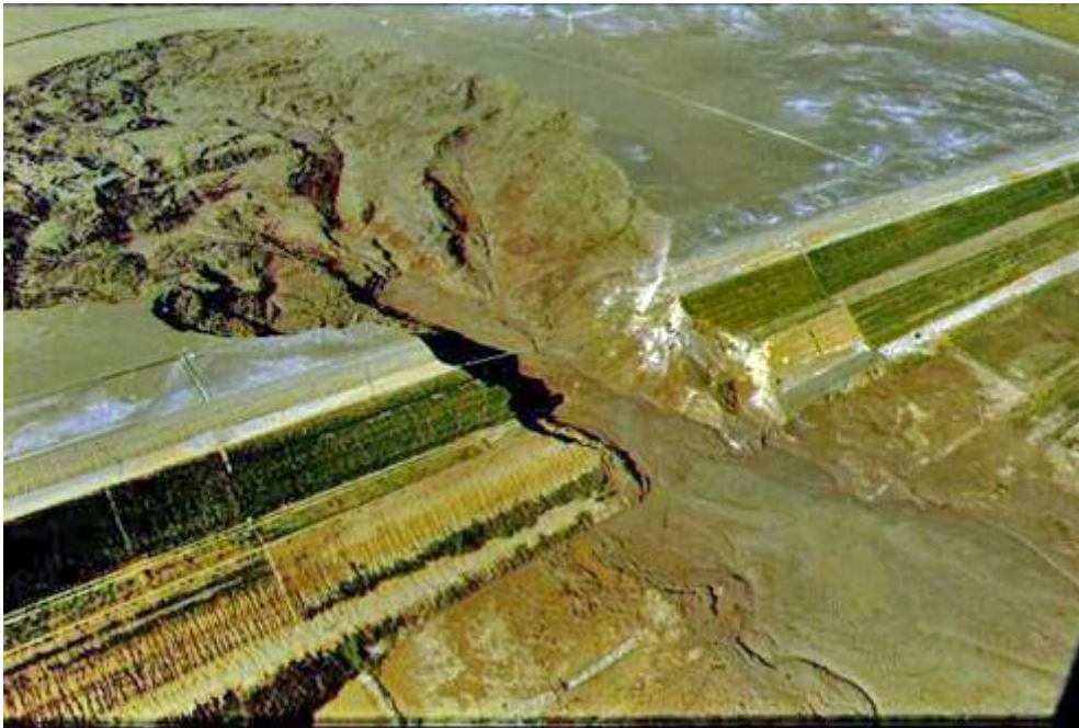
Figure 2-1. Aerial photograph of the Merriespruit tailings dam failure (after Minerals Council South Africa, 2020).
