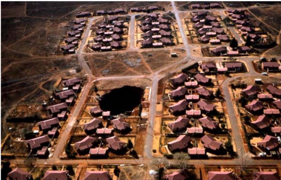
Fig. 5. The Blyvooruitzig Mine sinkhole that claimed six lives when mine employees houses were engulfed by subsidence in Carletonville, South Africa, in 1964 (Greyling, 2019).
