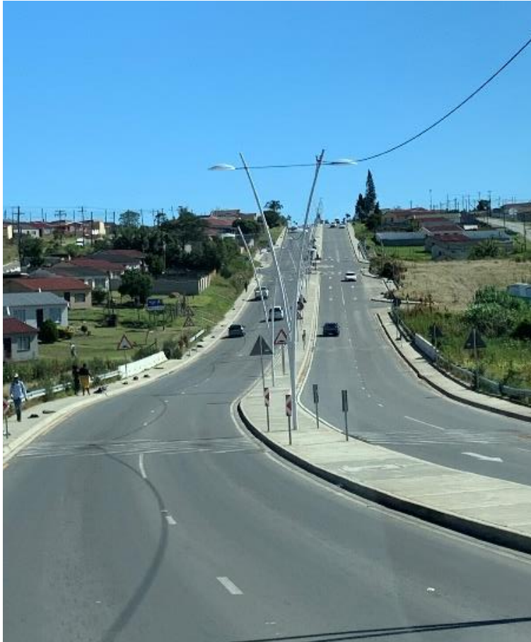
Figure 7.8 Lack of planted trees along the recently completed Qumza Public Transport Corridor.
