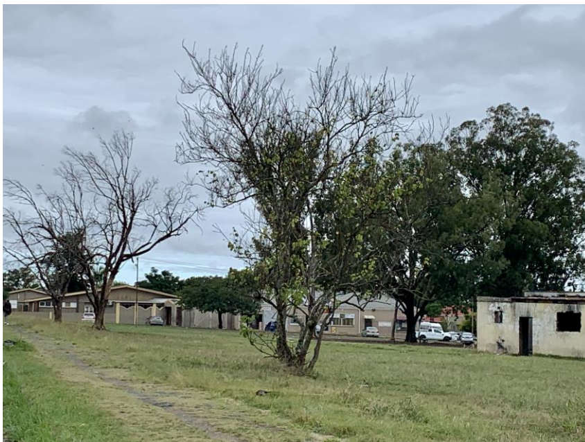
Figure 7.11 Vandalism of a municipal building located in the Camilla Park in the Qonce Inner City. Source: Author (2021)
