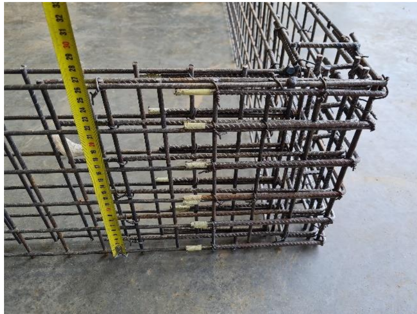
Figure 3-4: Joint reinforcing for proper moment transfer.
