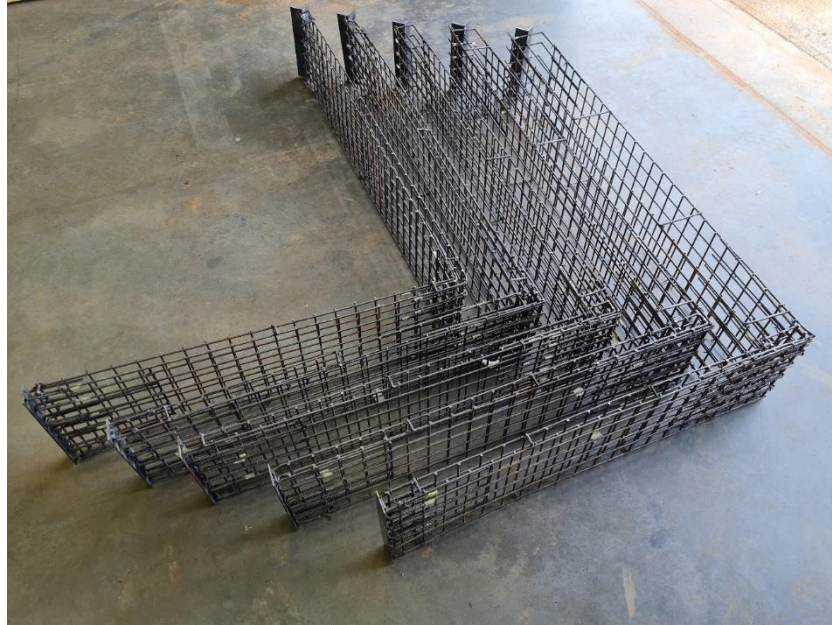
Figure 3-3: Steel reinforcement layout for the abutment specimens.
