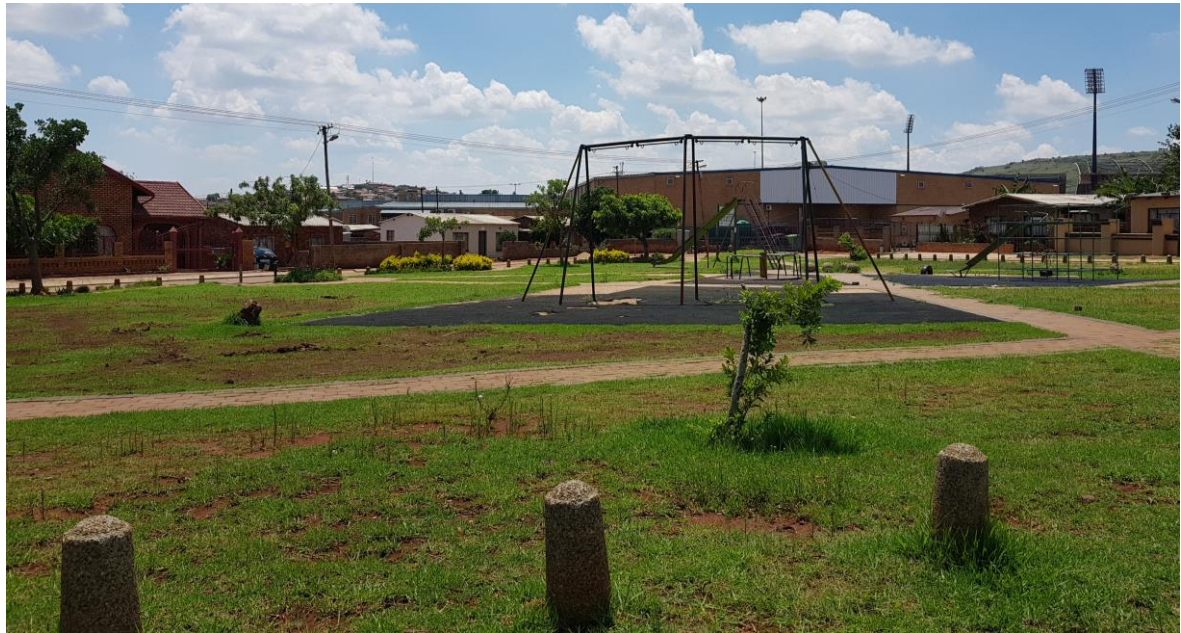
Figure 24: A park with worn surfaces and damaged play infrastructure
