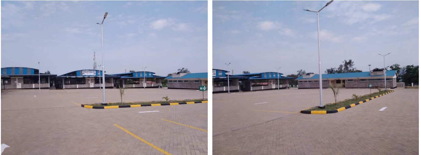
Plate 4.13: Completed market shades, ablution block at Uhuru Business Park.
