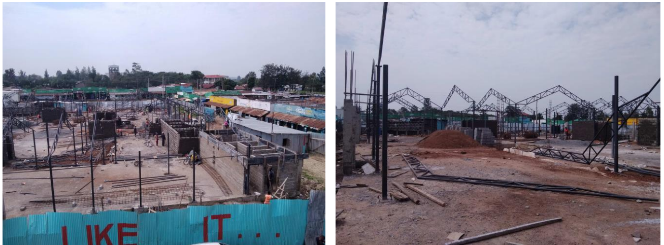
Plate 4.14: Ongoing construction of market shades at Otonglo Market
