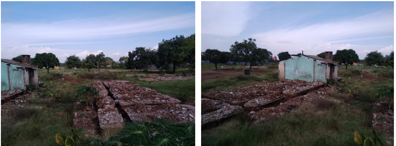
Plate 4.16: Existing bare land after flattening of all the units at Anderson Estate
