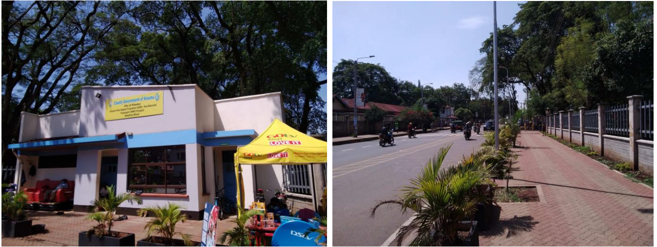
Plate 4.1: Newly constructed public toilet along Ang’awa Avenue with concrete planters in front and cabro paved pedestrian walkway along the boundary wall fence of rehabilitated Jaramogi Oginga Sports Ground.
