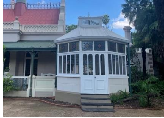
Figure 32: Conservatory from the front of the house.
