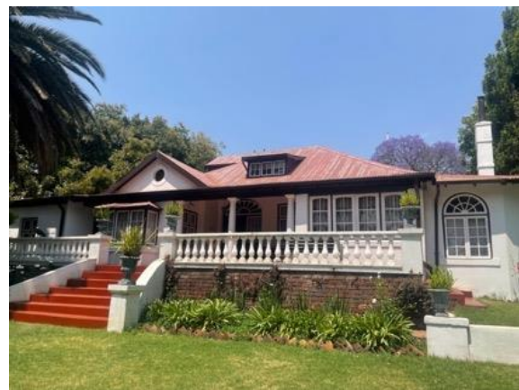
Figure 2: Front view of the Lindfield Victorian House Museum.
