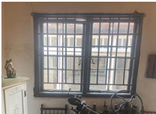
Figure 3: Barred windows of the servant's hall.
