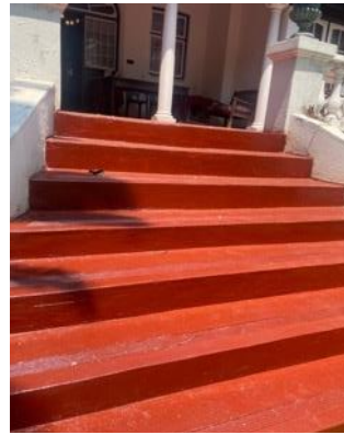
Figure 40: The patio was recently repainted.
