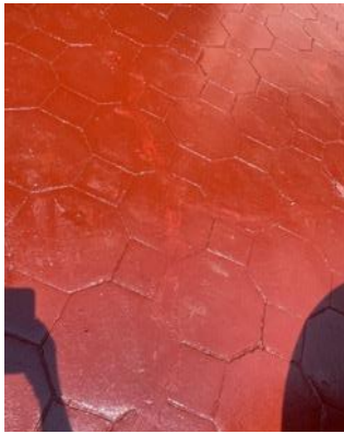
Figure 39: Recent repair of cracks on the patio.
