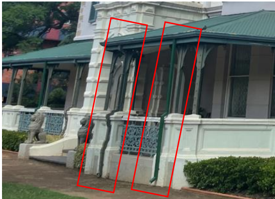
Figure 19: Old gutter (left) and new gutter (right) on front of house.
