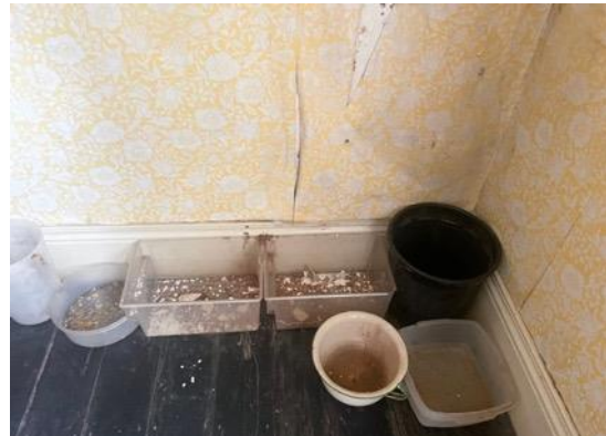
Figure 4: Degradation of the wall can be seen here through the eroded brick material.
