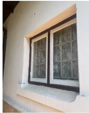
Figure 2: Barred windows of the dressing room.
