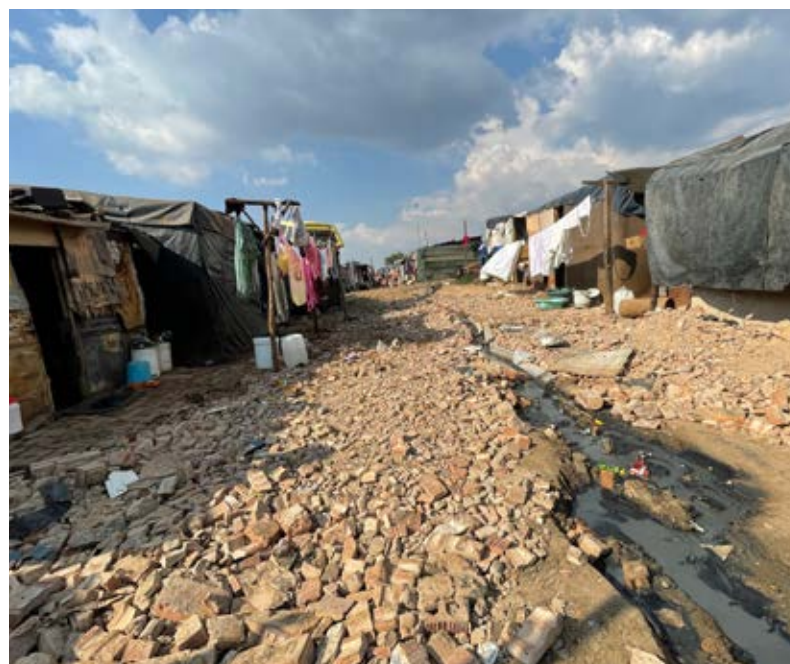
Figure 4.6. Loose Brick (Author 2022)
