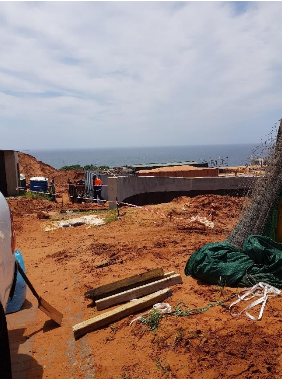
Figure 11: Local site undergoing residential construction.
